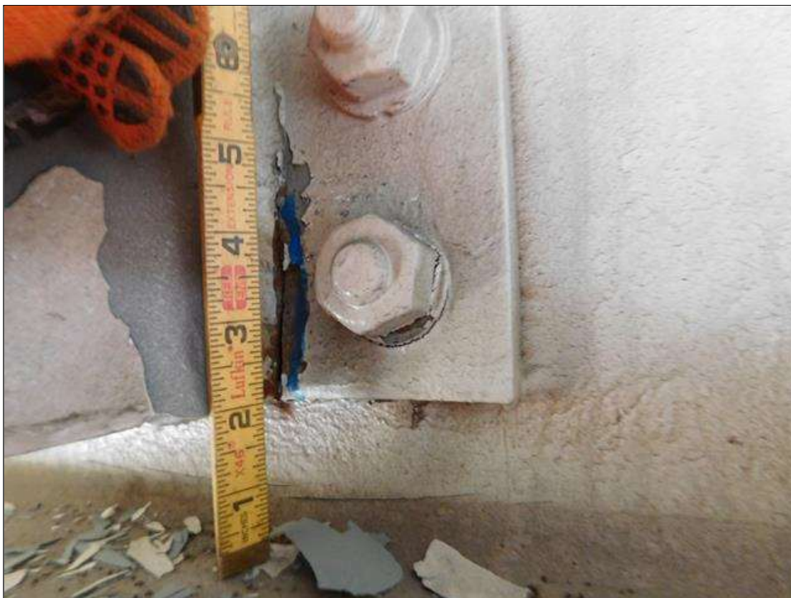
DIAPHRAGM 1 BAY 1 SPAN 2 CRACK IN BASE OF DIAPHRAGM 3" LONG X 1/16" WIDE
