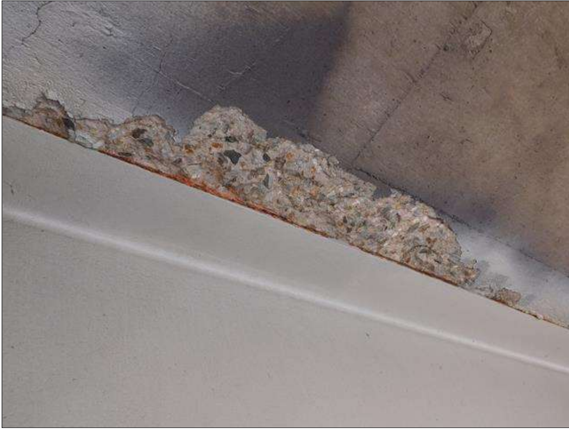
Span 3 Beam 3: SPALL AT EAST SIDE OF TOP FLANGE OF BEAM 3 SPAN 3. 3' LONG AT 12' FROM INTERIOR BENT 2. SPALL. SPALL AT EAST SIDE OF TOP FLANGE OF BEAM 3 SPAN 2. 2' LONG AT 20' FROM INTERIOR BENT 2
