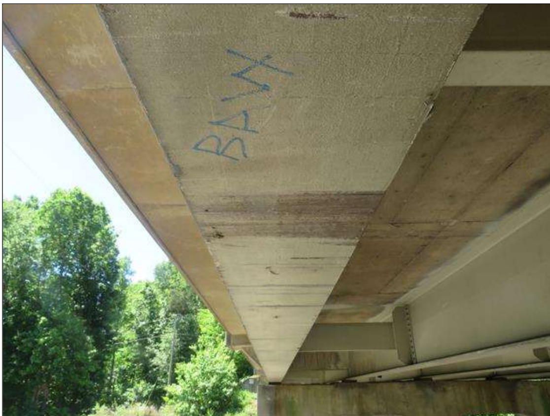
Span 3 Beam 5: SUPPLEMENTAL INSPECTION IMPACT DAMAGE 2022.: two 1/4in deep indentions in bottom flange of beam 5 span 3 at 16.5ft from bent 2 for a length of 1ft . SCATTERED SCRAPES
