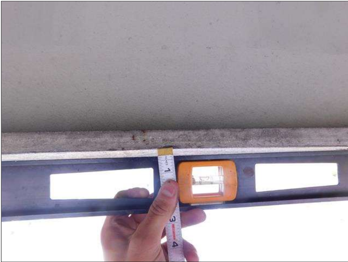
Span 3 Beam 2: BEAM 2 SPAN 3 DEFLECTED UPWARD 1/2" AT 19.5" FROM INTERIOR BENT 2 FOR A LENGTH OF 4', WITH SCRAPES ON BOTTOM FLANGE
