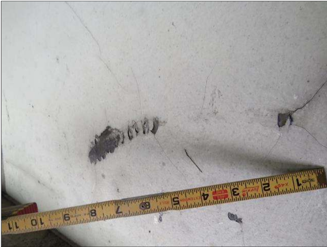
Span 3 Beam 1: SUPPLEMENTAL INSPECTION IMPACT DAMAGE 2022.: POINT OF IMPACT 9' LONG WITH SCATTERED 1" DEEP INDENTIONS THROUGH OUT BOTTOM FLANGE , AT 12'-9" OUT FROM INT. BENT 3 . BEAM 1 DEFLECTION 1" TO THE WEST. TOP FLANGE PULLED LOOSE FROM BEAM EAST SIDE FOR A LENGTH OF 30' X 3/4" .,EAST SIDE OF BOTTOM FLANGE BENT UPWARD 1/2in. SCATTERED SCRAPES ALONG BOTTOM FLANGE AND WEB(PAR) . SCATTERED OLD SCRAPES AND INDENTIONS ALONG BOTTOM FLANGE .
