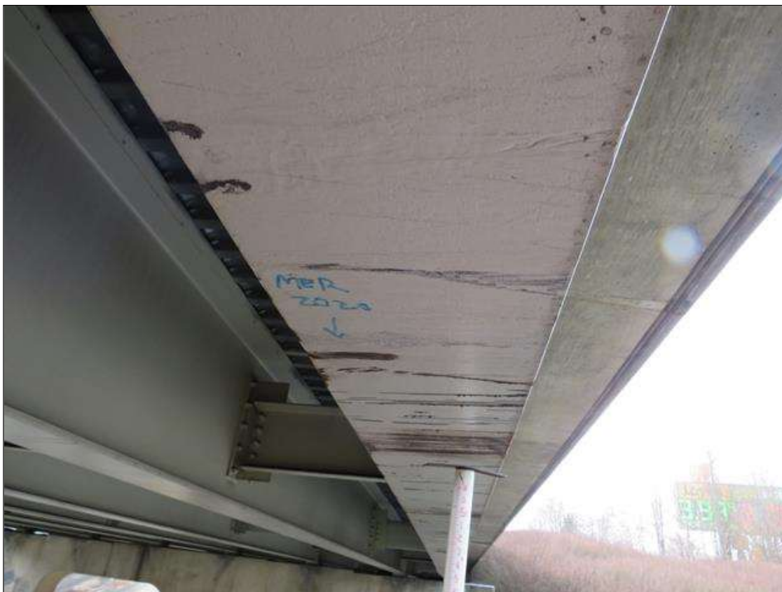
Span 2 Beam 1: SCATTERED SCRAPES
