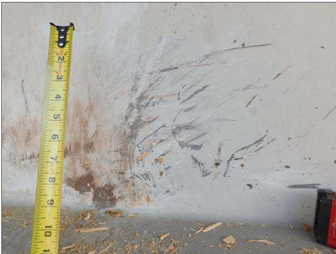
SPAN 2 BEAM 1: SCATTERED SCRAPES IN LEFT SIDE OF BOTTOM WEB
