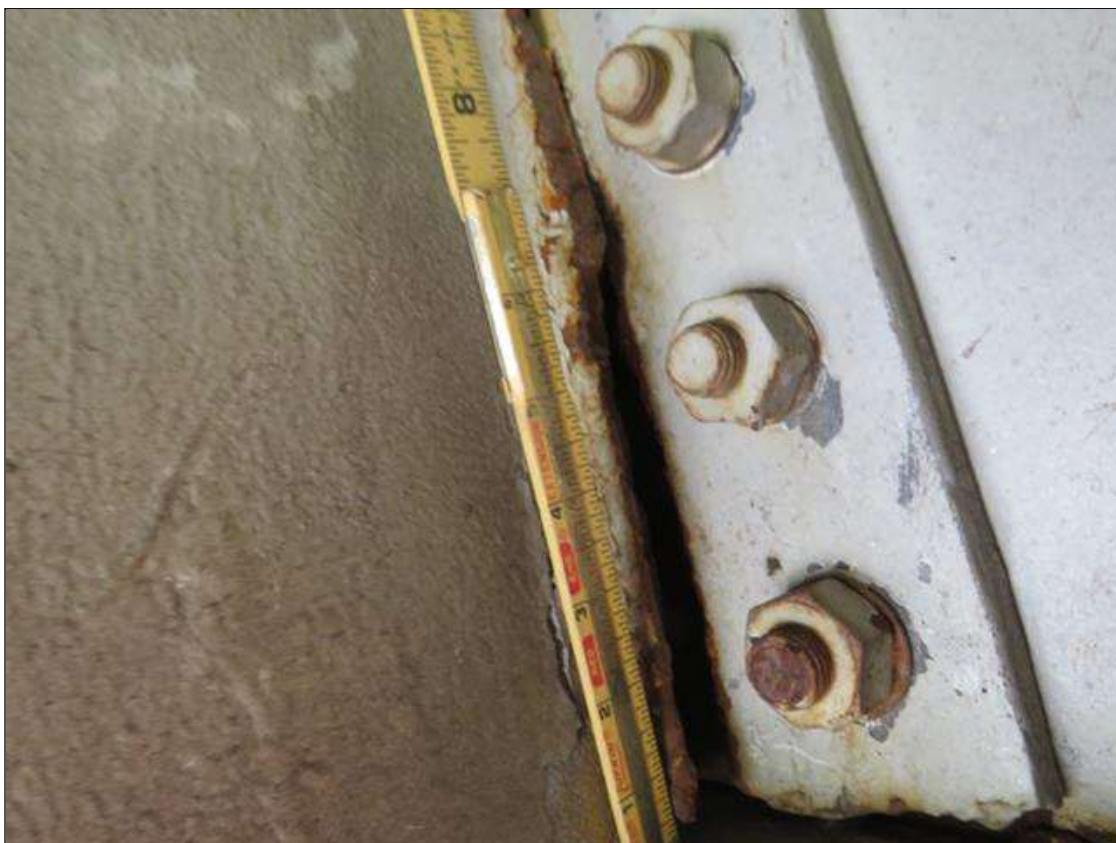
UP TO 1" WIDE CRACKING DIAPHRAGM 2 BAY 1
