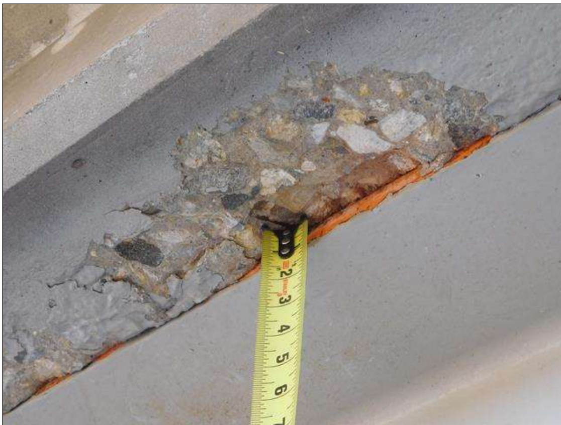
SCATTERED POPOUTS IN BOTTOM DECK AT LEFT SIDE OF BEAM 1 AT BOTTOM FLANGE
