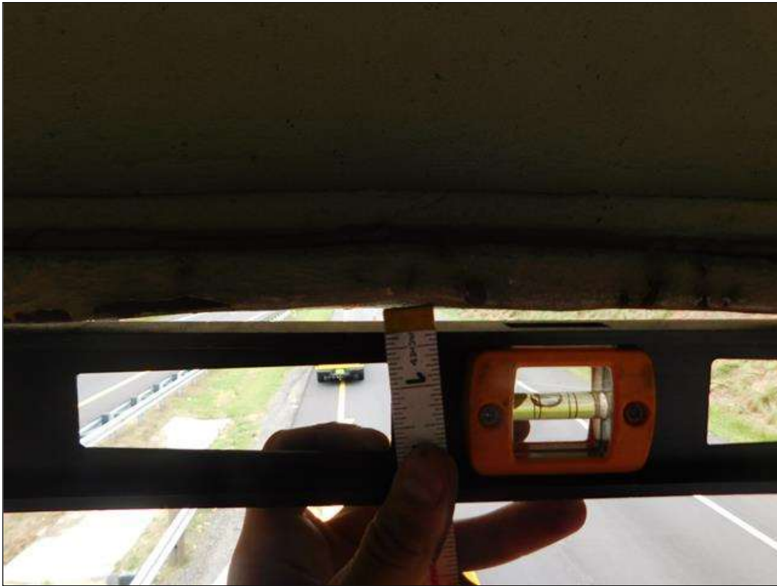
Span 3 Beam 1: BEAM 1 SPAN 3 HAS INDENTION AT 21.167' FROM INTERIOR BENT 2 FOR A LENGTH OF 2', WITH UPWARD DEFLECTION OF 1/2". ONE INDENTION 15.5' FROM INTERIOR BENT 2 FOR A LENGTH OF 1', WITH UPWARD DEFLECTION OF 1/4"
