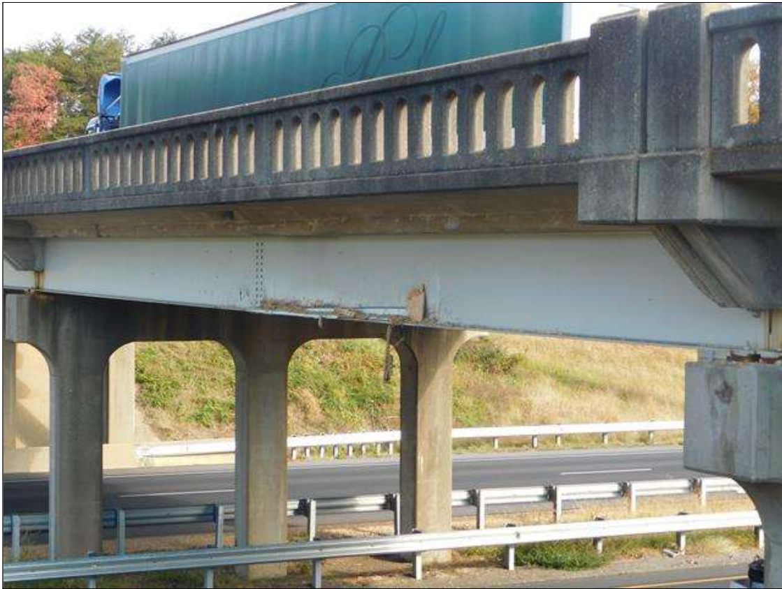
SPAN 2 BEAM 1: OVERVIEW OF IMPACT DAMAGE TO BEAM 1 (PAR)
