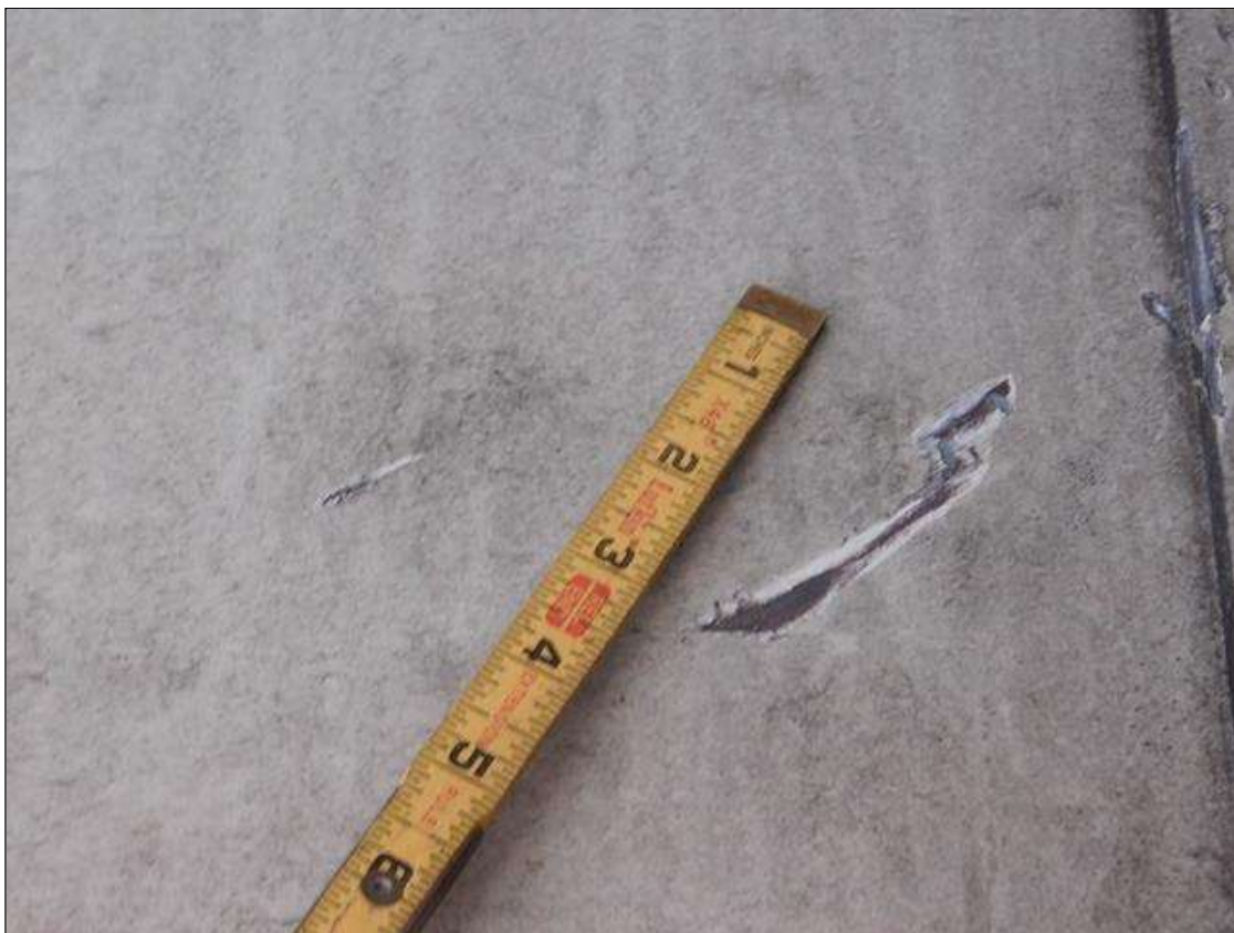
BEAM 3 SPAN 1 SCATTERED SCRAPES ALONG THE WEB OF BEAM 3
