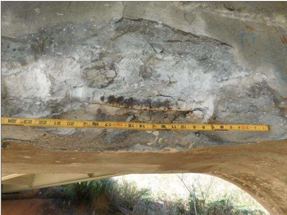
INT. BENT 1 CAP SPALLING BENEATH BEAM 3 AT THE BOTTOM OF CAP 3'-3" LONG X 11" HIGH X 8" DEEP WITH 1 REINFORCING BAR EXPOSED (PAR)
