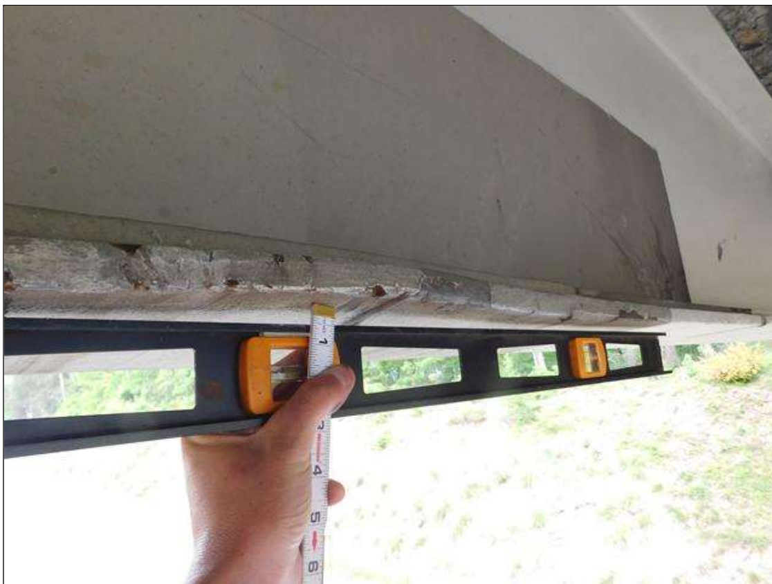
Span 3 Beam 1: BEAM 1 SPAN 3 DEFLECTED UPWARD 1/2" AT 22.75' FROM INTERIOR BENT 2 FOR A LENGTH OF 1'
