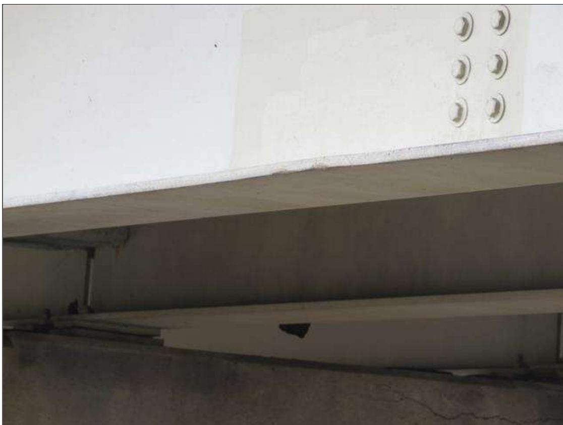
Span 3 Beam 5: SUPPLEMENTAL INSPECTION IMPACT DAMAGE 2022.: two 1/4in deep indentions in bottom flange of beam 5 span 3 at 16.5ft from bent 2 for a length of 1ft
