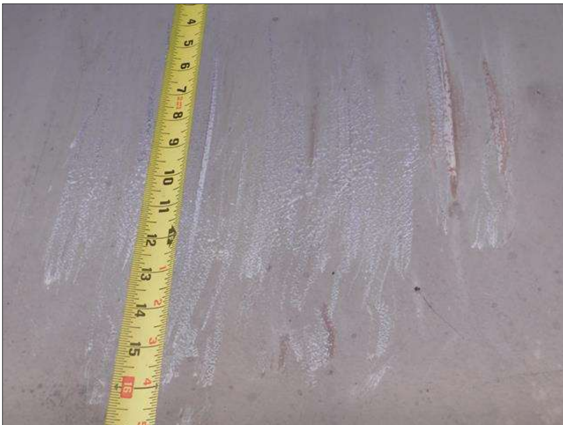
Span 2 Beam 4: SCATTERED SCRAPES TO LEFT SIDE OF WEB.
