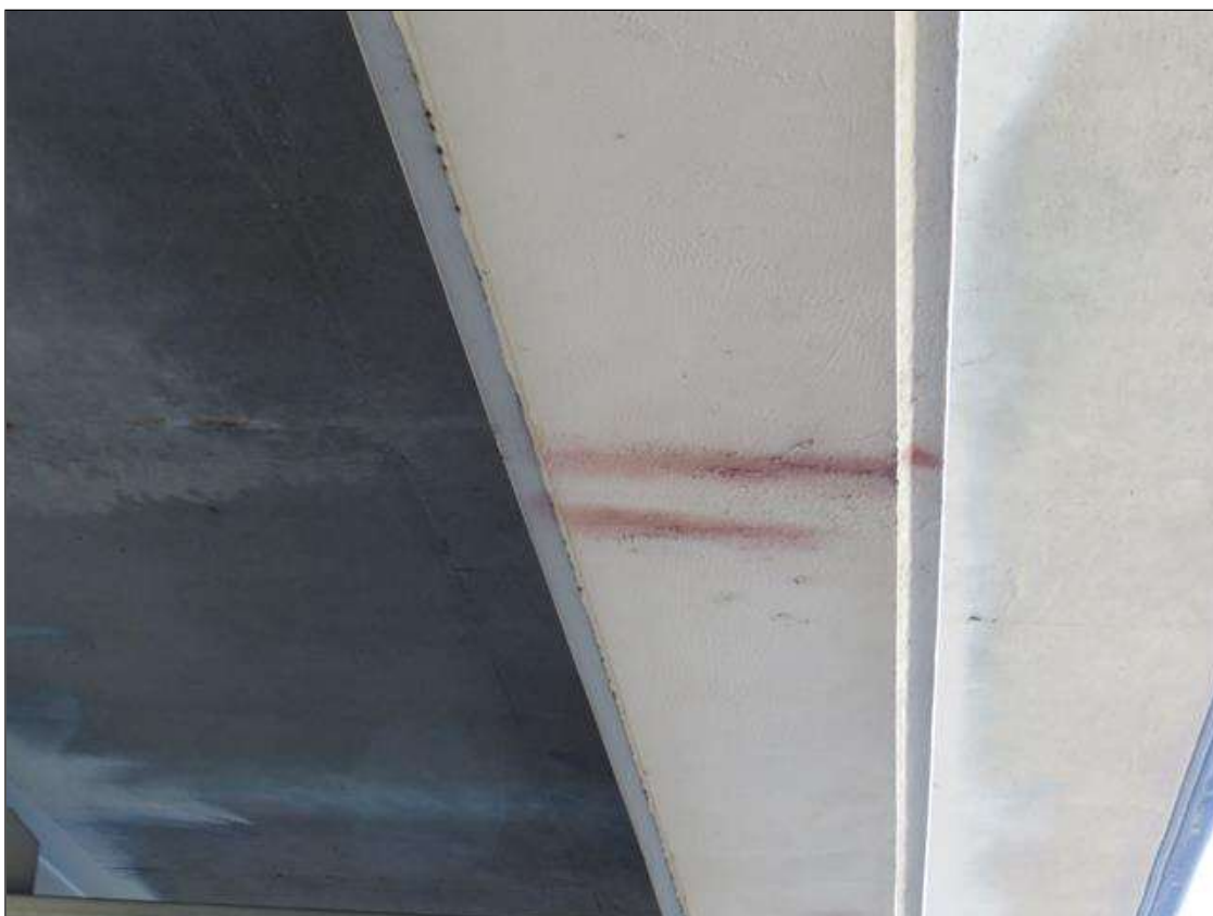
Span 3 Beam 1: SUPPLEMENTAL INSPECTION IMPACT DAMAGE 2021 :scattered scrapes
