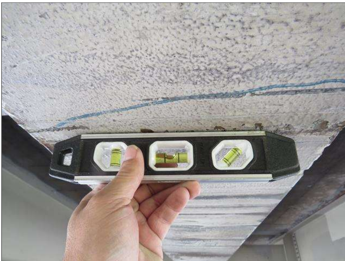
Span 3 Beam 2: SUPPLEMENTAL INSPECTION IMPACT DAMAGE 2022.: beam 2 span 3 deflected upward 1/2in at 19.5in from bent 2 for a length of 4ft, with scrapes on bottom flange . SCATTERED SCRAPES ALONG THE WEB .
