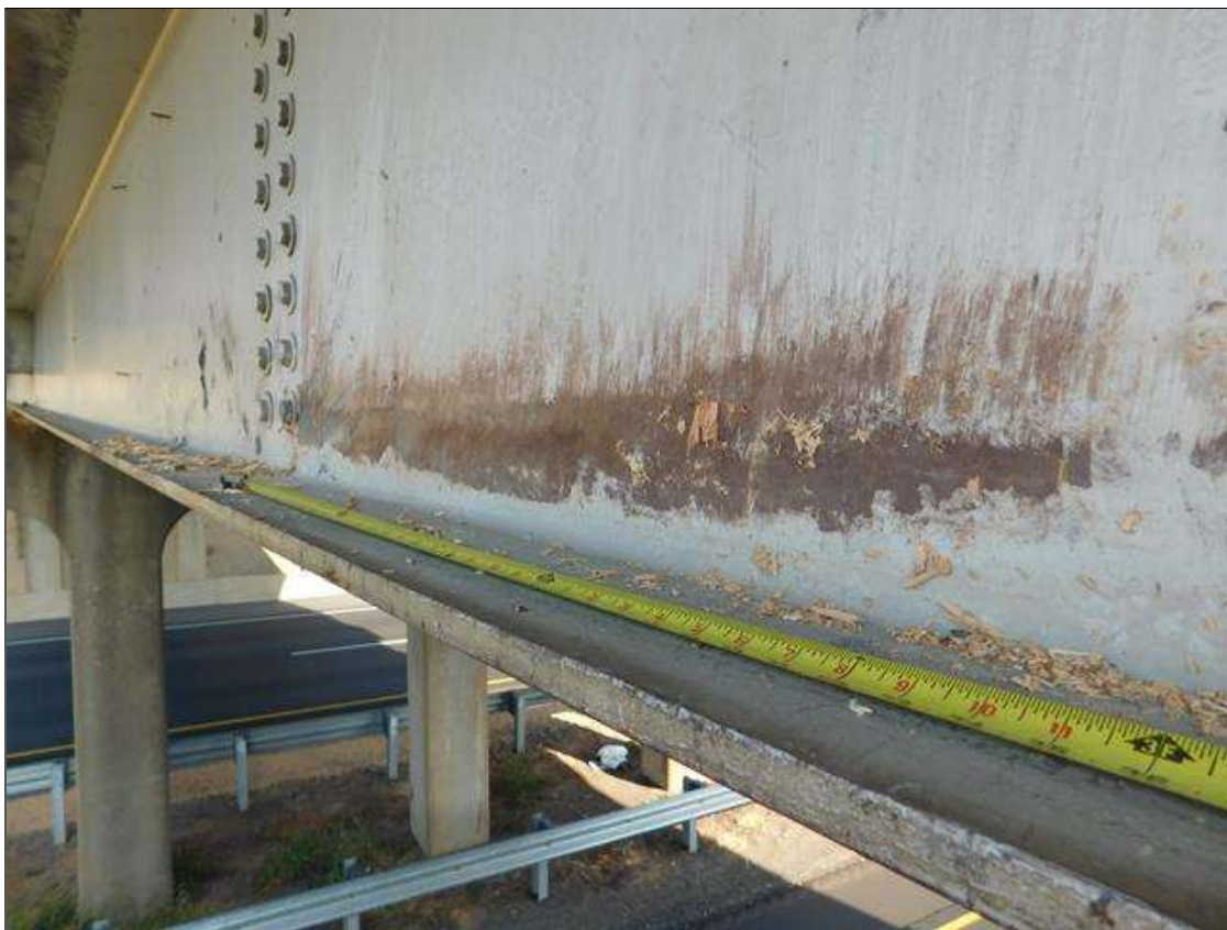
SPAN 2 BEAM 1: SCATTERED SCRAPES TO BOTTOM WEB
