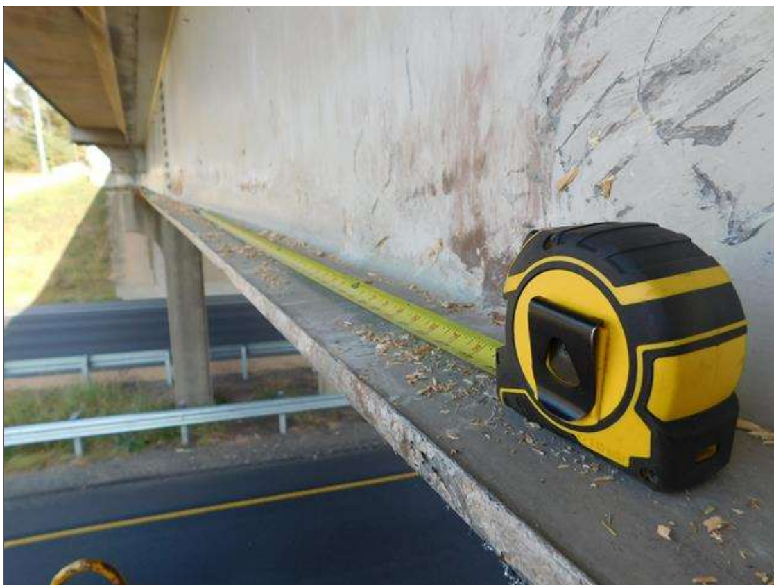
Span 2 Beam 1: POINT OF IMPACT TO BEAM 1 AT 24'8" FROM INT. BENT 1 FOR A LENGTH OF 15'.
