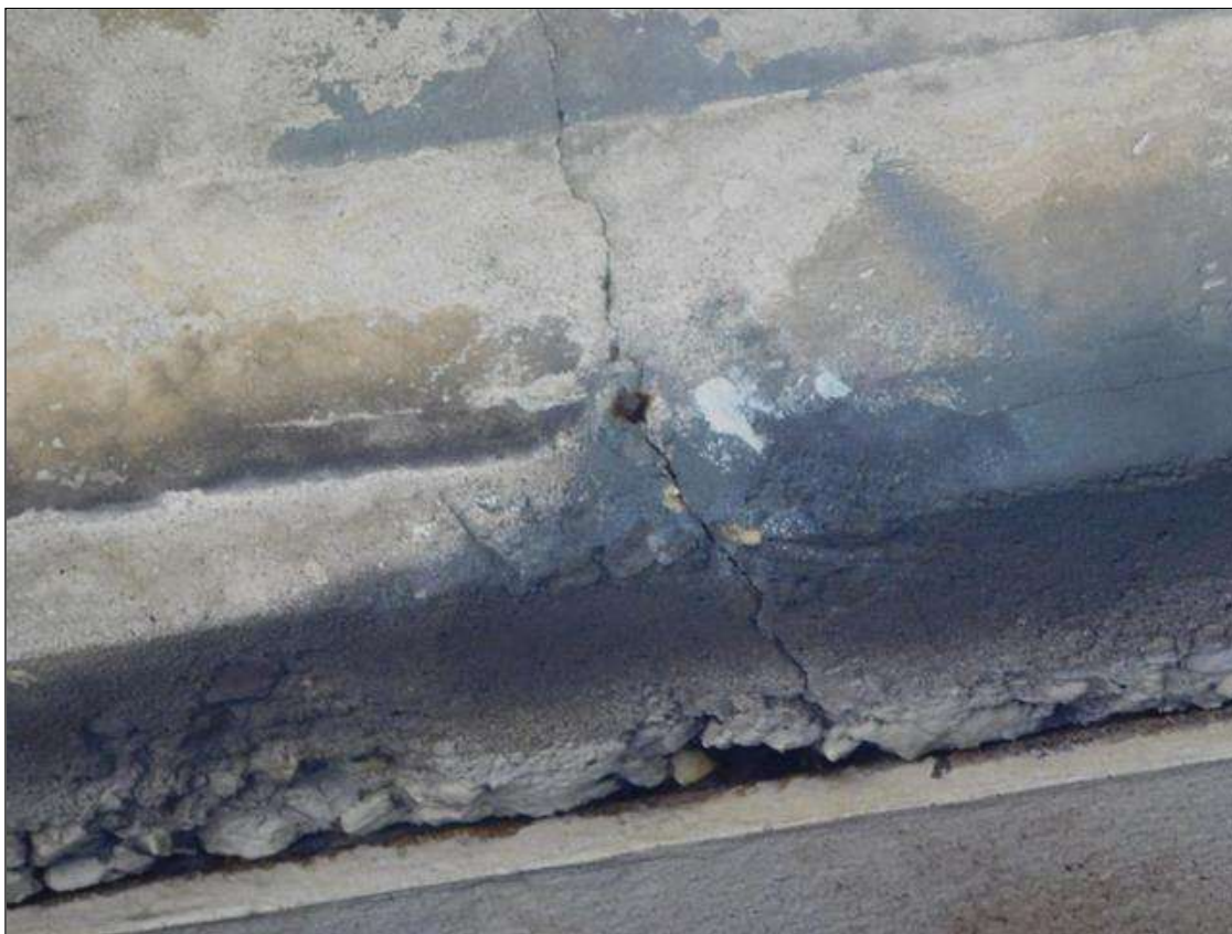
Span 2 Deck: SUPPLEMENTAL INSPECTION 2021 : THERE ARE 2 HAIRLINE CRACK IN THE RIGHT OVERHANG ABOVE POINT OF IMPACT
