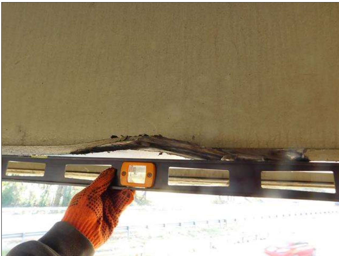
BEAM 2 SPAN 2 POINT OF IMPACT 20" LONG X BOWED UPWARD 1 1/2" LEFT FLANGE AT 4'-3" OUT FROM INT. BENT 1
