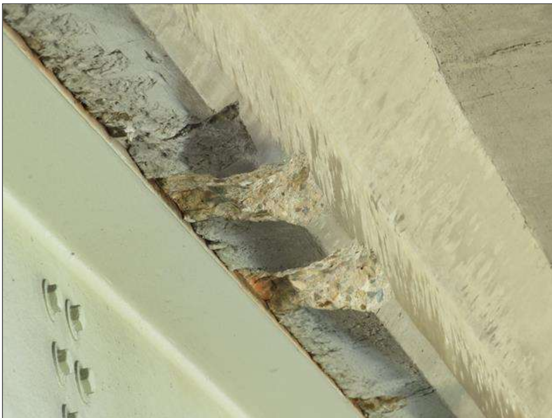
Span 3 Deck: SUPPLEMENTAL INSPECTION IMPACT DAMAGE 2022.surface spalling up to 1/2in deep, full length, underside of deck along both sides of beam 1.
