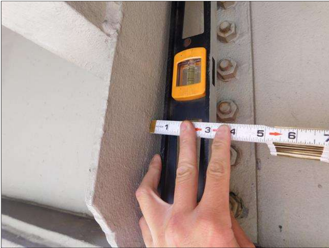
BEAM 1 SPAN 3: DIAPHRAGM 2 BAY 2 DEFLECTED SOUTHWARD FOR 1/2"
