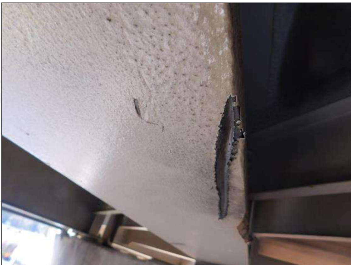
BEAM 2 SPAN 1 , 12" LONG X 1/16" DEEP SCRAPES ALONG THE BOTTOM FLANGE OF BEAM
