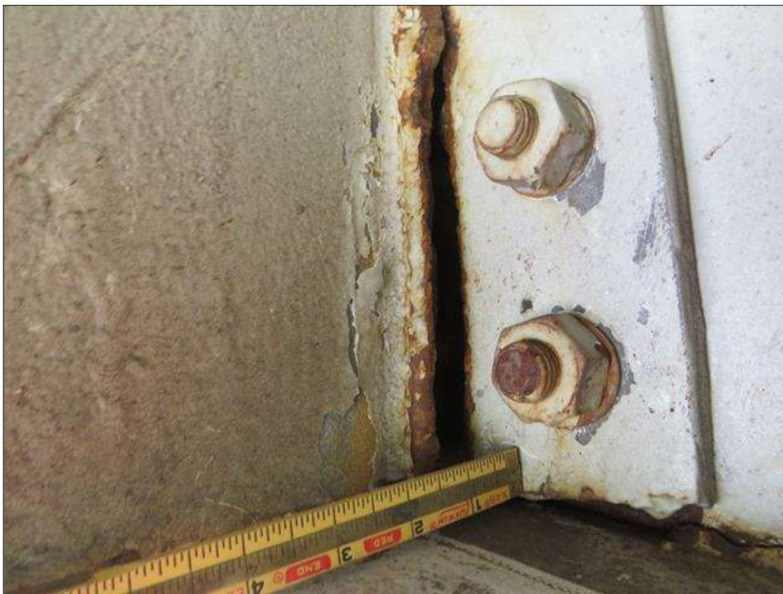
UP TO 1" WIDE CRACKING DIAPHRAGM 2 BAY 1
