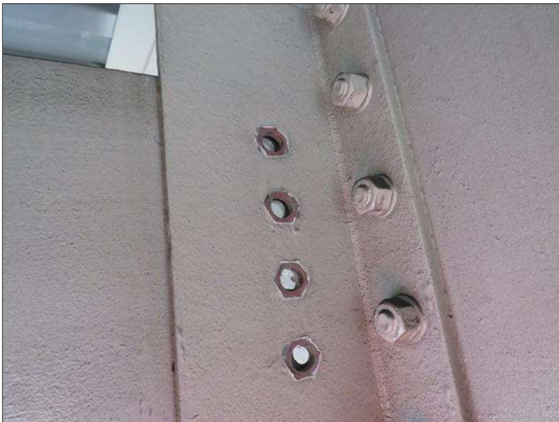
SPAN 2 BAY 1 DIAPHRAM 2 ALL 4 BOLTS MISSING AT DIAPHRAM ATTACHMENT TO BEAM 1 (PAR)
