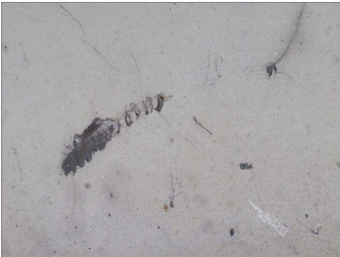
Span 3 Beam 2: SUPPLEMENTAL INSPECTION IMPACT DAMAGE 2022.: SCATTERED SCRAPES WEB OF BEAM 2 .
