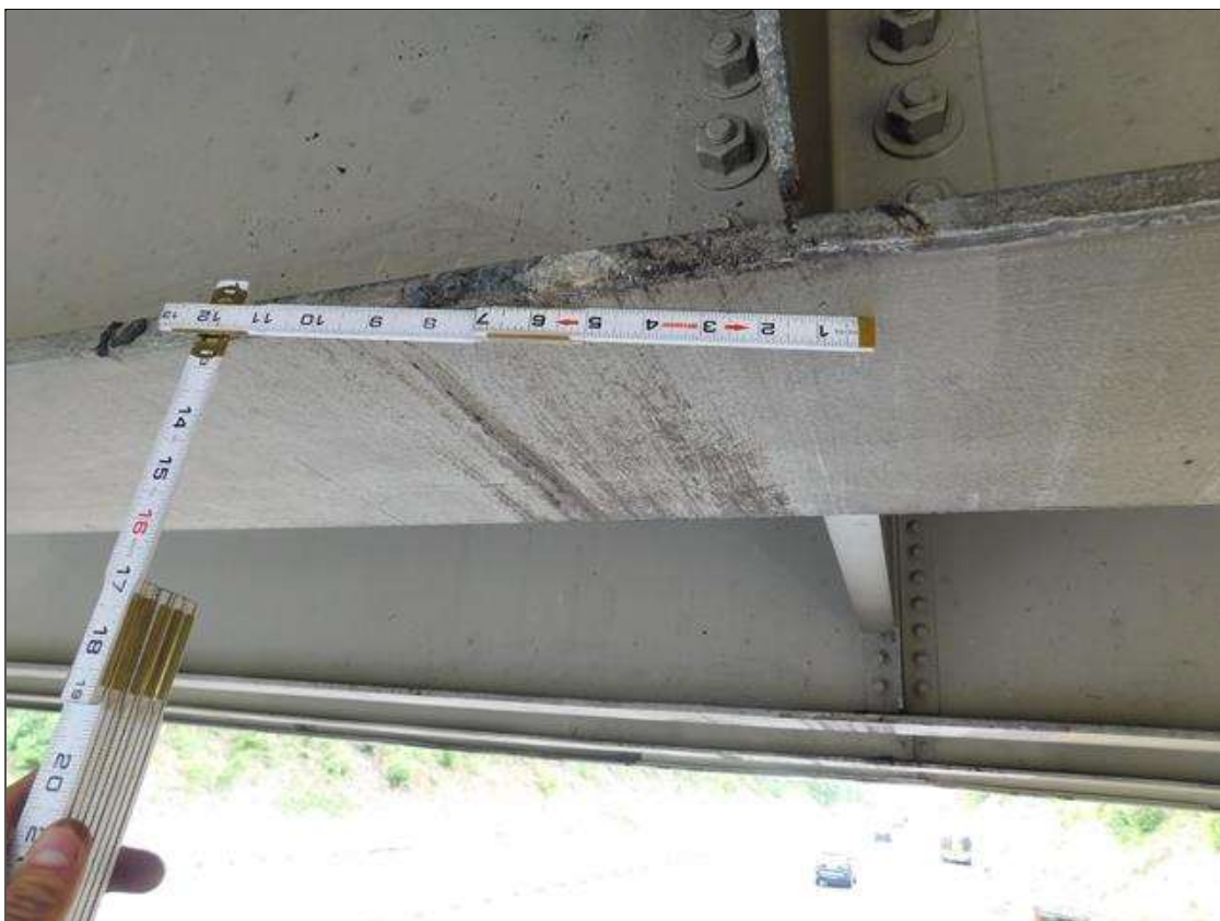
Span 3 Beam 4: BEAM 4 SPAN 3 HAS SCRAPES TO BOTTOM FLANGE AT 16.75' FROM INTERIOR BENT 3 FOR A TOTAL LENGTH OF 1'
