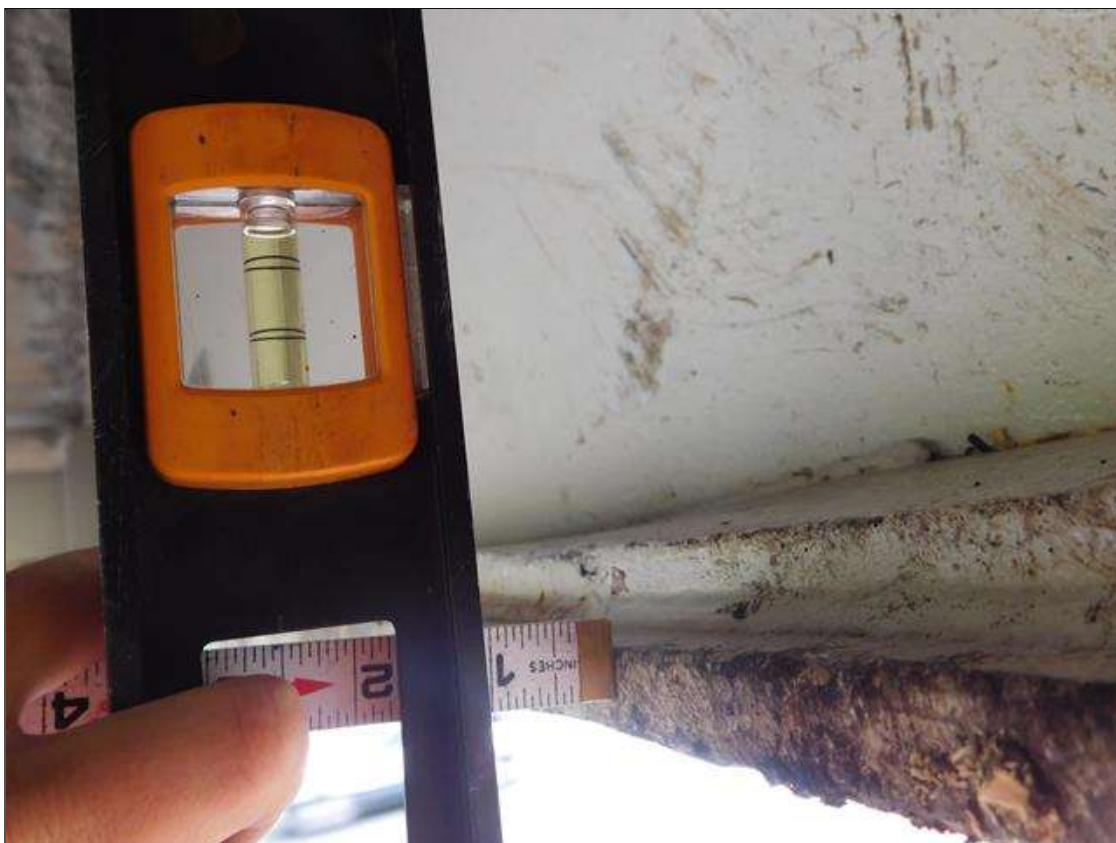
Span 3 Beam 1: BEAM 1 SPAN 3 IS DEFLECTED WESTWARD 1" FOR A TOTAL LENGTH OF 10'. PAR
