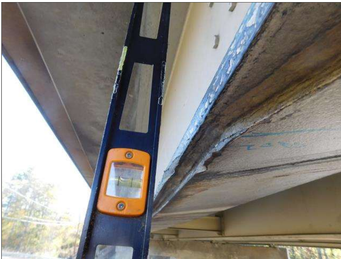
BEAM 1 SPAN 2 BEAM SWEEP EASTWARD 1 1/2" (PAR)
