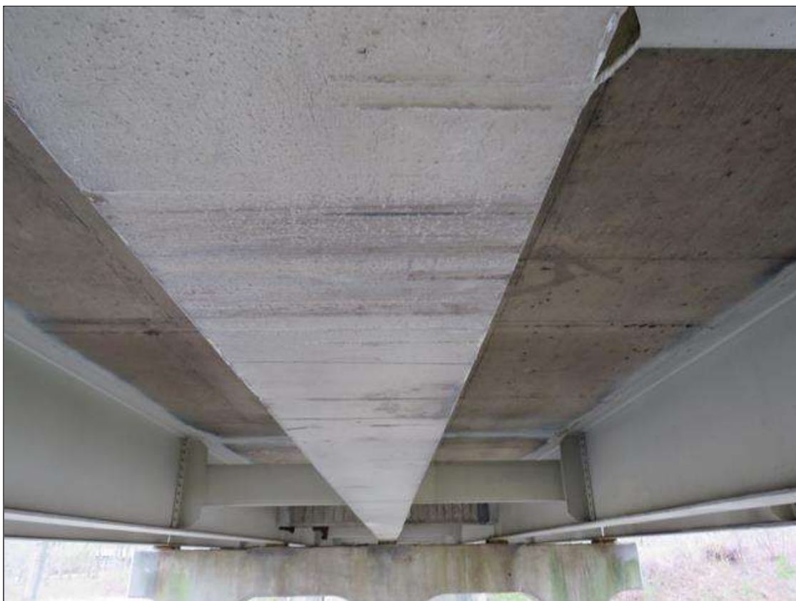
Span 3 Beam 3: SUPPLEMENTAL INSPECTION IMPACT DAMAGE 2022. : SCATTERED SCRAPES ALONG BOTTOM FLANGE OF BEAM 3
