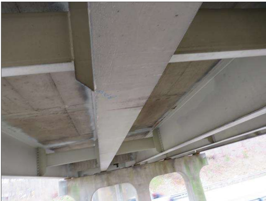
Span 3 Beam 4: bSUPPLEMENTAL INSPECTION IMPACT DAMAGE 2022.: Beam 4 Span 3 has scrapes to bottom flange at 16.75ft from bent 3 for a total length of 1ft
