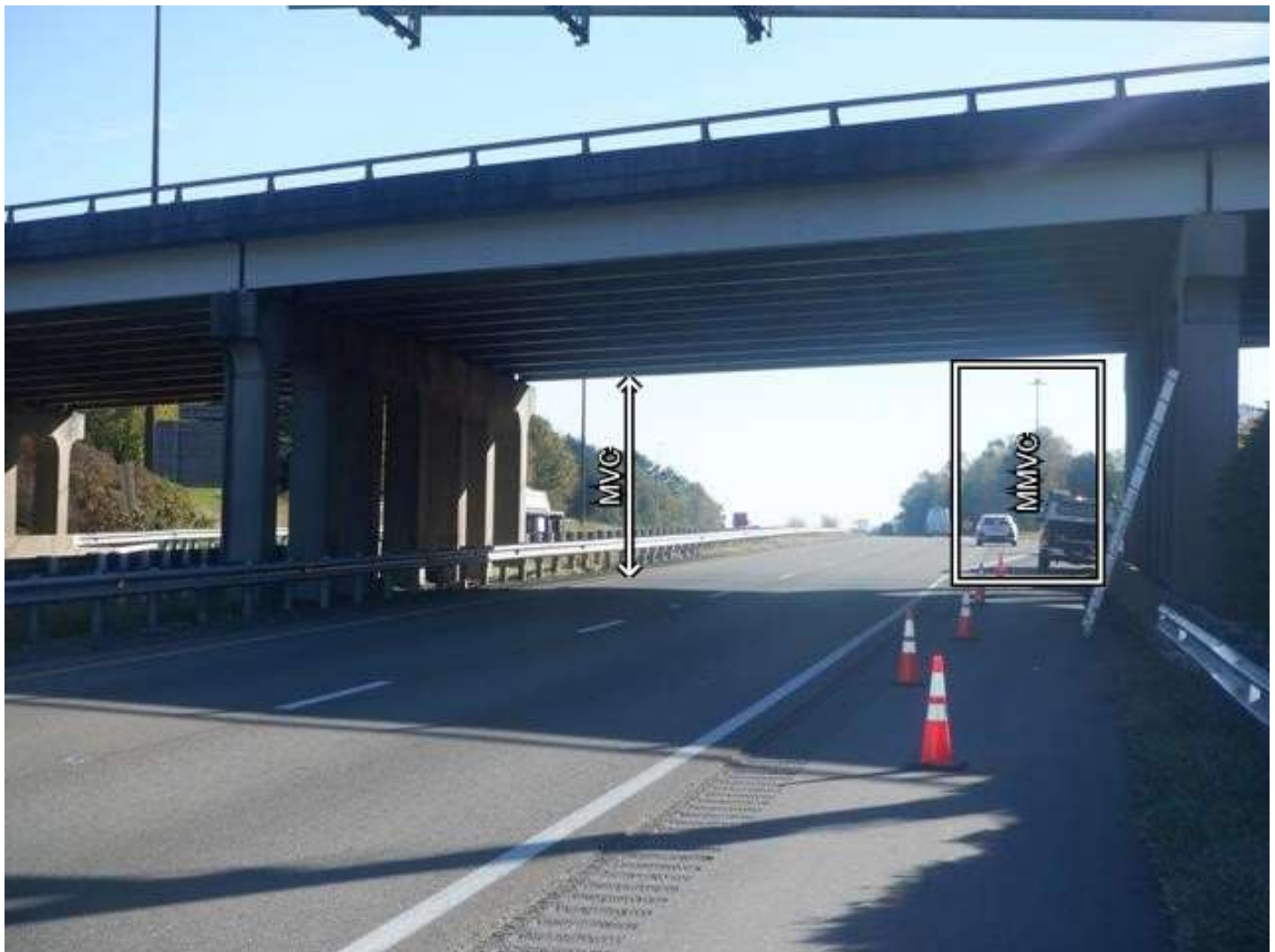
vertical clearance looking East Span 2 (choose 1)
