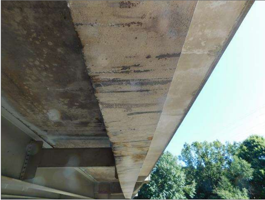
Span 2 Beam 5: 2021 SUPPLEMENTAL INSPECTION 2021 : BEAM 5 SPAN 2 POINT OF IMPACT 10" LONG X 1" HIGH AT 14'10" OUT FROM INT. BENT 2 , WITH THE BEAM BEING SWEEPED EAST WARD UP TO 3" .SCATTERED SCRAPES ALONG THE BOTTOM FLANGE . PREVIOUS IMPACT DAMAGE AS NOTED IN THE ADDITIONAL COMMENTS SECTION. (PAR)
