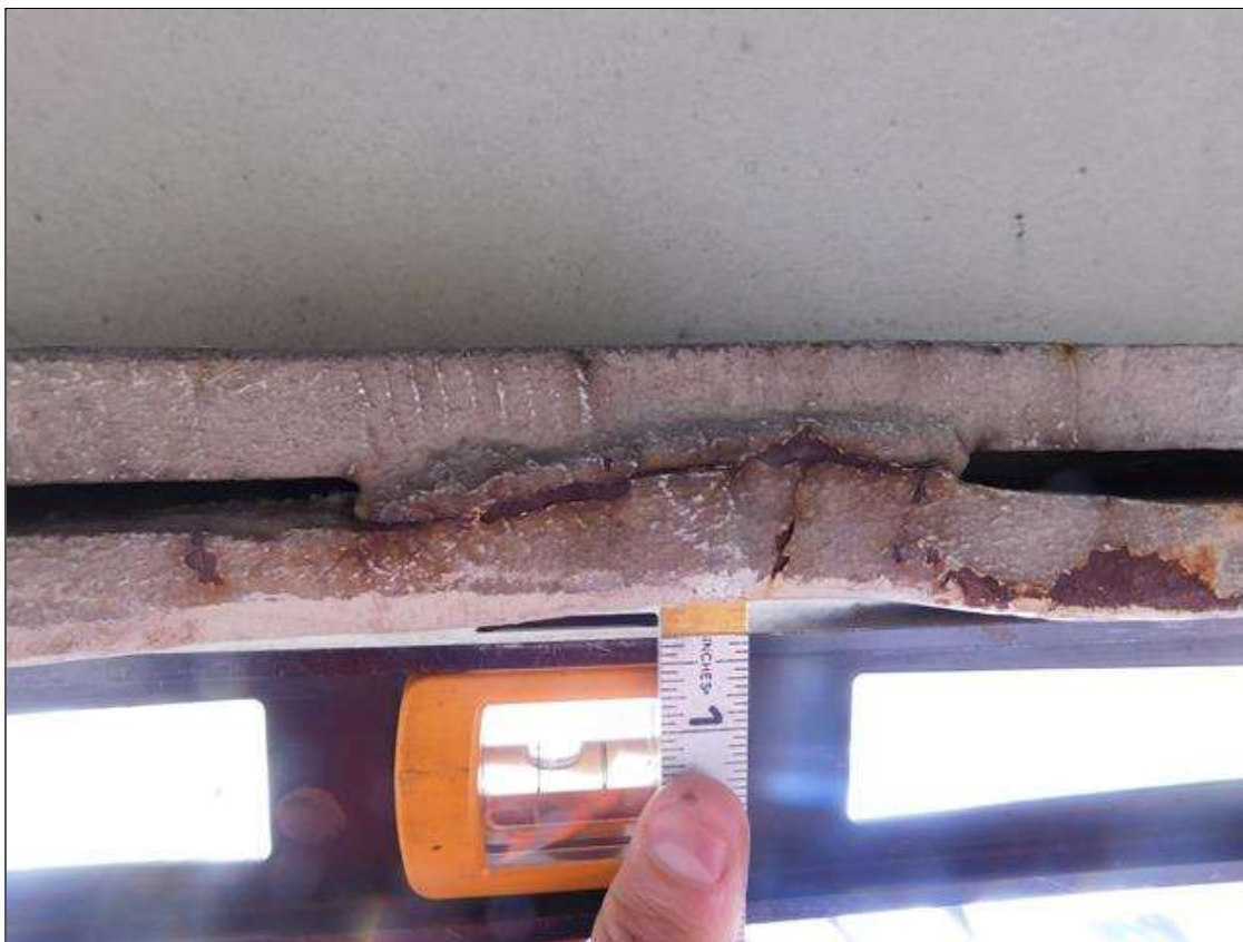
Span 3 Beam 1: BEAM 1 SPAN 3 HAS INDENTATION AT 21.167' FROM INTERIOR BENT 2 FOR A LENGTH OF 2', WITH UPWARD DEFLECTION OF 1/2". ONE INDENTION 15.5' FROM INTERIOR BENT 2 FOR A LENGTH OF 1', WITH UPWARD DEFLECTION OF 1/4"
