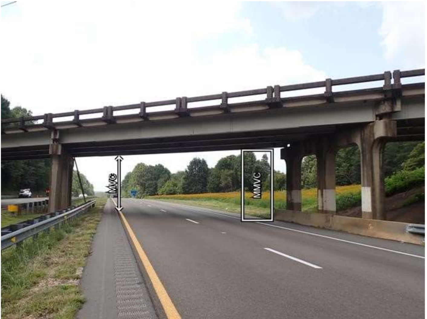
span 3 vertical clearance looking West
