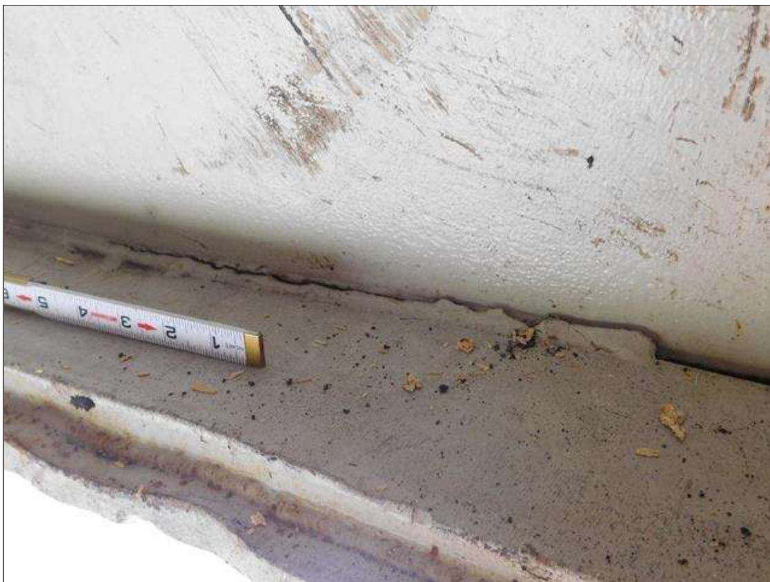
Span 3 Beam 1: CRACK IN WELD OF PLATE AT BOTTOM FLANGE OF BEAM 1 SPAN 3 MEASURED AT 17' FROM INTERIOR BENT 3 FOR A LENGTH OF 1'
