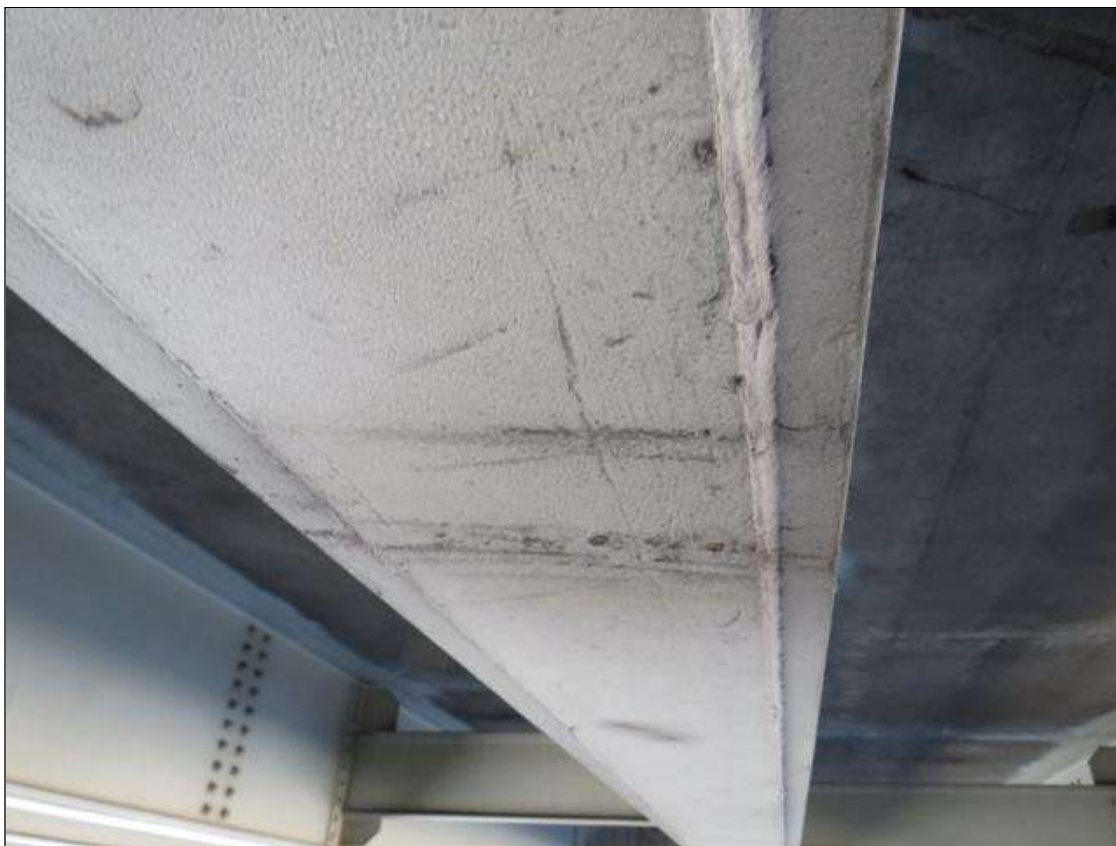
Span 3 Beam 4: SUPPLEMENTAL INSPECTION IMPACT DAMAGE 2021: scattered scrapes
