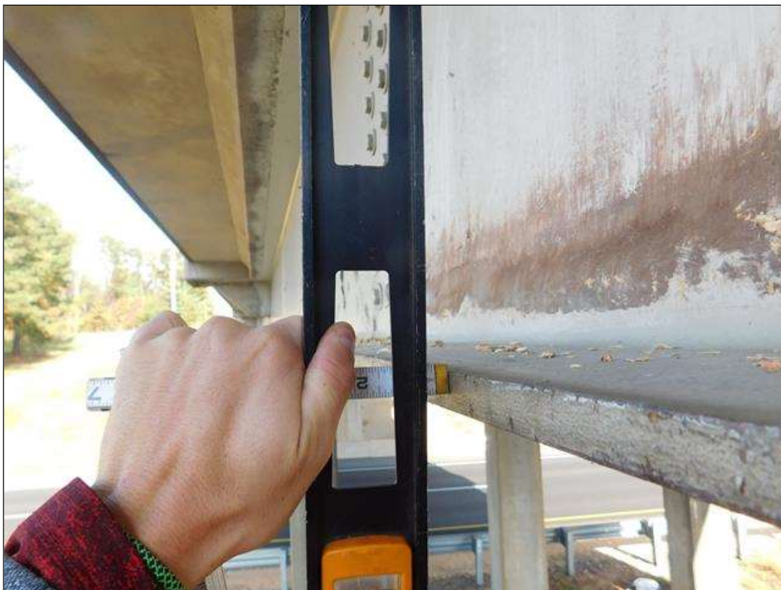
SPAN 2 BEAM 1: BEAM 1 SWEEPED EASTWARD 1" FOR A LENGTH OF 20' (PAR)
