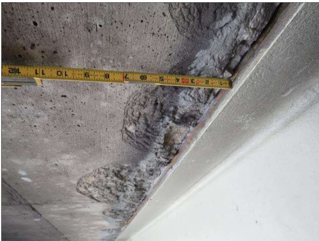
Span 3 Deck: SUPPLEMENTAL INSPECTION IMPACT DAMAGE 2022.surface spalling up to 1/2in deep, full length, underside of deck along both sides of beam 2.
