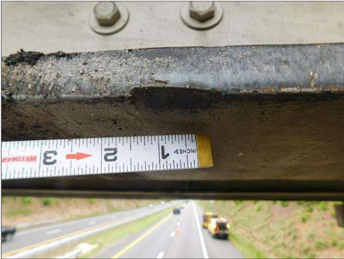
Span 3 Beam 5: BEAM 5 SPAN 3 HAS SCRAPES ON BOTTOM FLANGE AT 16.5' FROM INTERIOR BENT 3 FOR A TOTAL LENGTH OF 1'. INDENTATION AT 16.417' FROM INTERIOR BENT 3, 1" LONG BY 1/4" DEEP
