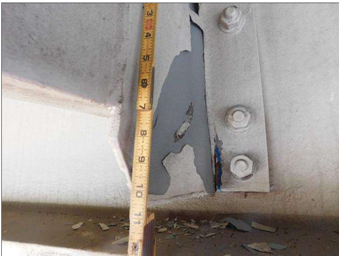
DIAPHRAGM 1 BAY 1 SPAN 2 BOWED
