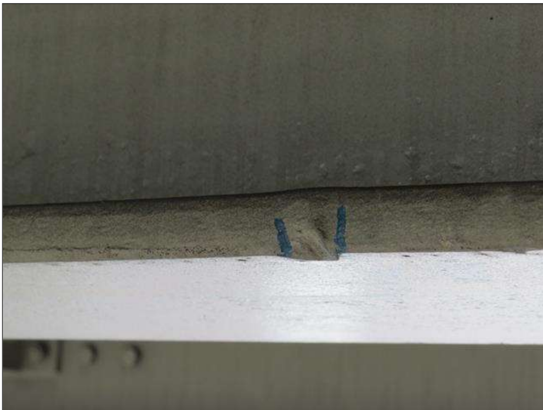
Span 2 Beam 2: 2022 OLD INDENTIONS BEAM 4
