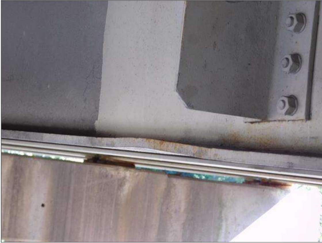
Span 2 Beam 2: SUPPLEMENTAL INSPECTION 2021: POINT OF IMPACT 8" LONG WITH A 1/2" DEEP GOUGE AT 18'-8" FROM INT. BENT 2 , WITH BEAM BEING SWEEPED EASTWARD 1/2". SCATTERED SCRAPES ALONG THE BEAM (PAR) THERE IS A BENT UP SECTION ON THE WEST BOTTOM FLANGE 4" LONG X 1" HIGH AT 20' OUT FROM INT. BENT 1 (PAR)
