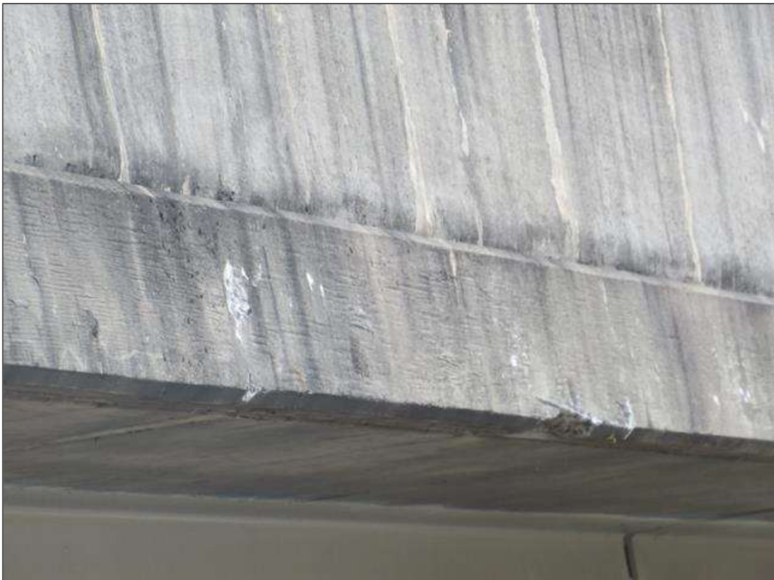
Span 2 LEFT RAIL SCATTERED INDENTIONS BOTTOM
