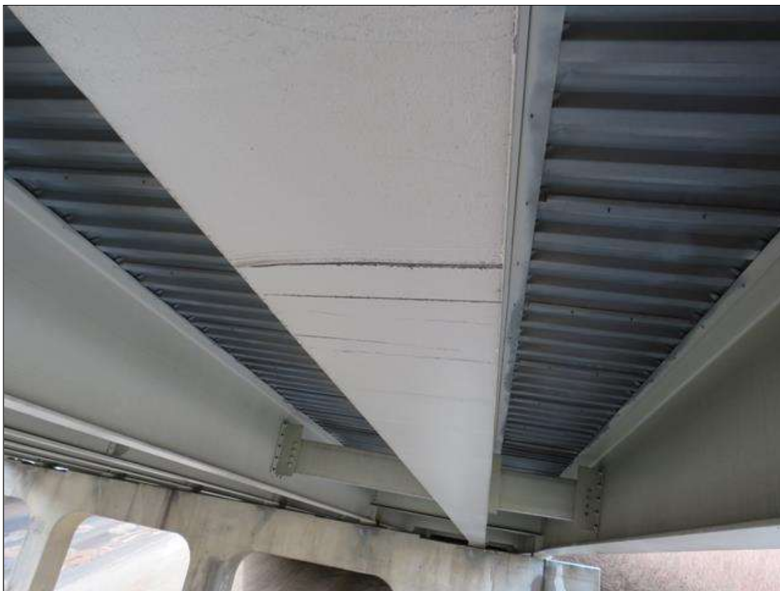
Span 2 Left Bridge Rail: 2022 SUPPLEMENTAL INSPECTION SCATTERED SCRAPES ON BEAM 2
