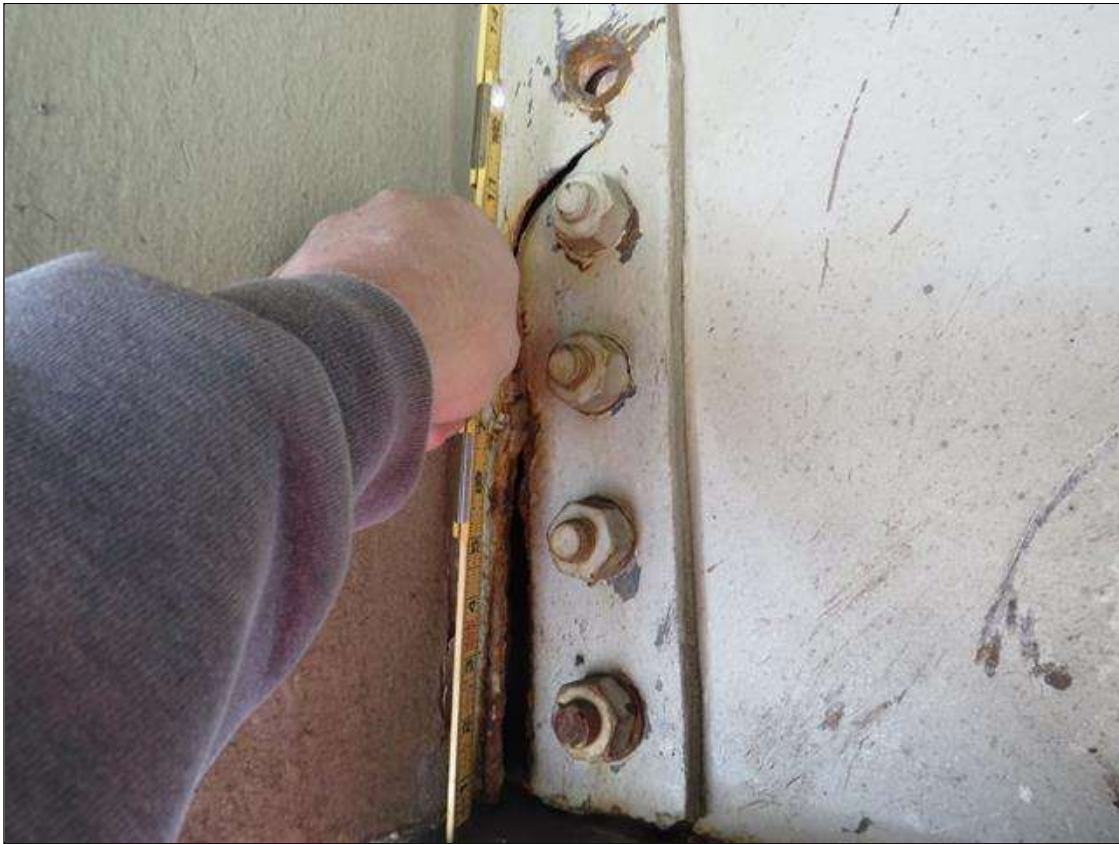
SUPPLEMENTAL INSPECTION IMPACT DAMAGE 2022: SPAN 3 DIAPHRAGM 2 BAY 1: 20 BOLTS WITH 6 MISSING ON BEAM 1, UP TO 1' HIGH CRACKING STRATING AT 1/32" WIDE AT TOP AND UP TO 1 1/8" AT BOTTOM OF DIAPHRAGM (PAR) .
