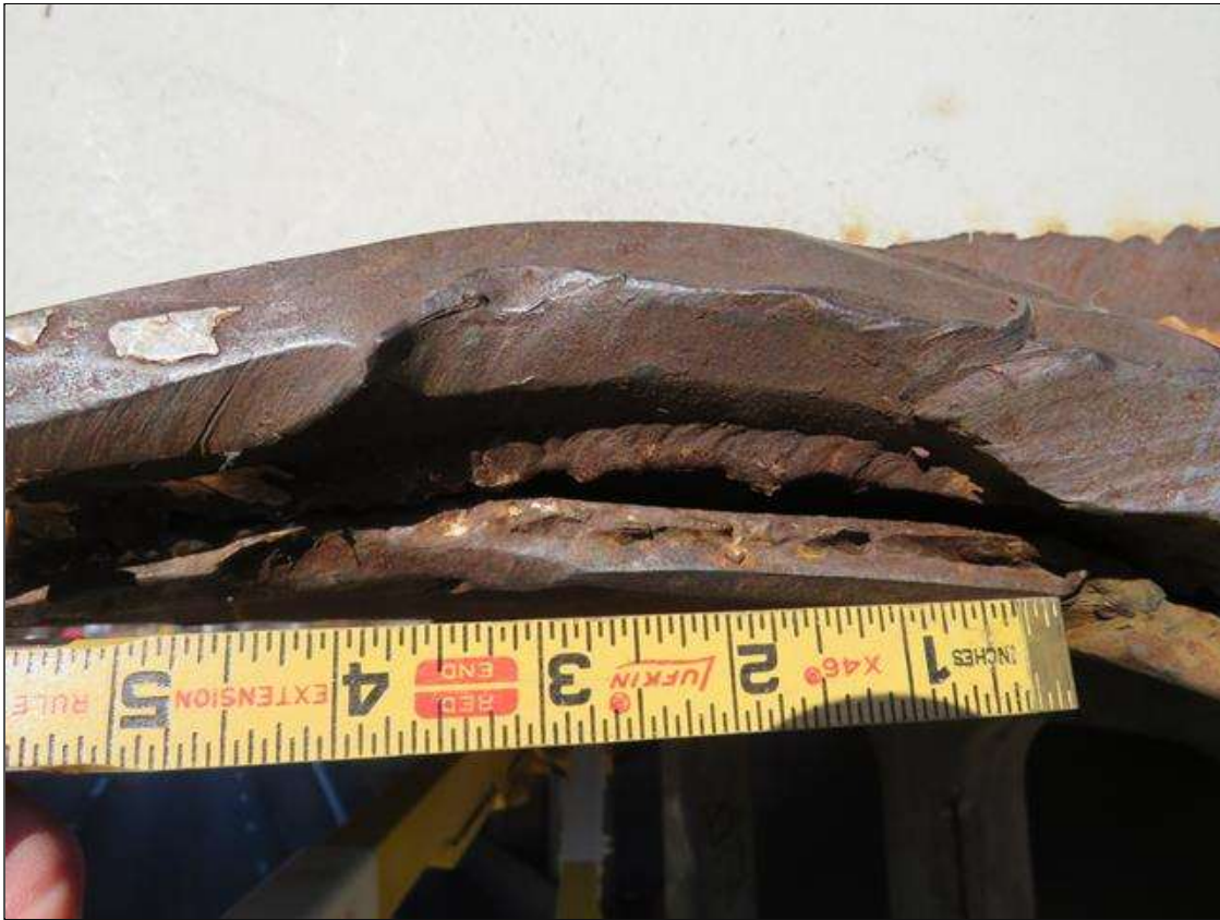
Span 3 Beam 11: SUPPLEMENTAL INSPECTION IMPACT DAMAGE 2021 area of previous impact damage, distortion of bottom flange vertical up to 2" lateral up to 1/2" with broken cover plate weld [10" long]. new area of impact damage 6" long x 2" high at 13'-5" out from int. bent 3 . with the bottom cover plate being broken loose from bottom flange 10" long x 2" deep . there are also two older 1/2" indentions in the same area . Beam 11 is swept westward up to 1 1/2". (par) there is a 2" diameter torch cut hole at both ends of of the 6' length .
