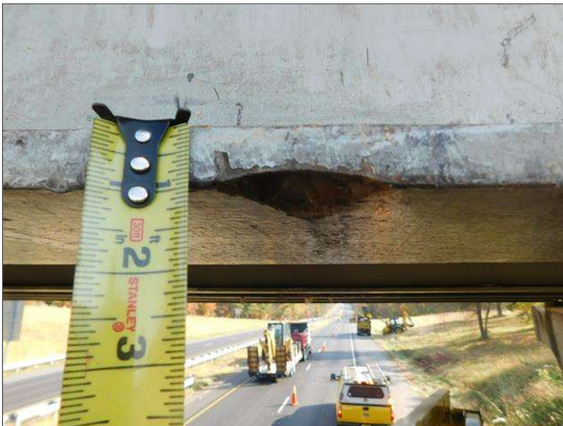
Span 2 Beam 1: INDENTION IN LEFT SIDE OF BOTTOM FLANGE AT 147" FROM INT. BENT 1, 2" LONG X 1" WIDE X 1/8" DEEP (PAR)
