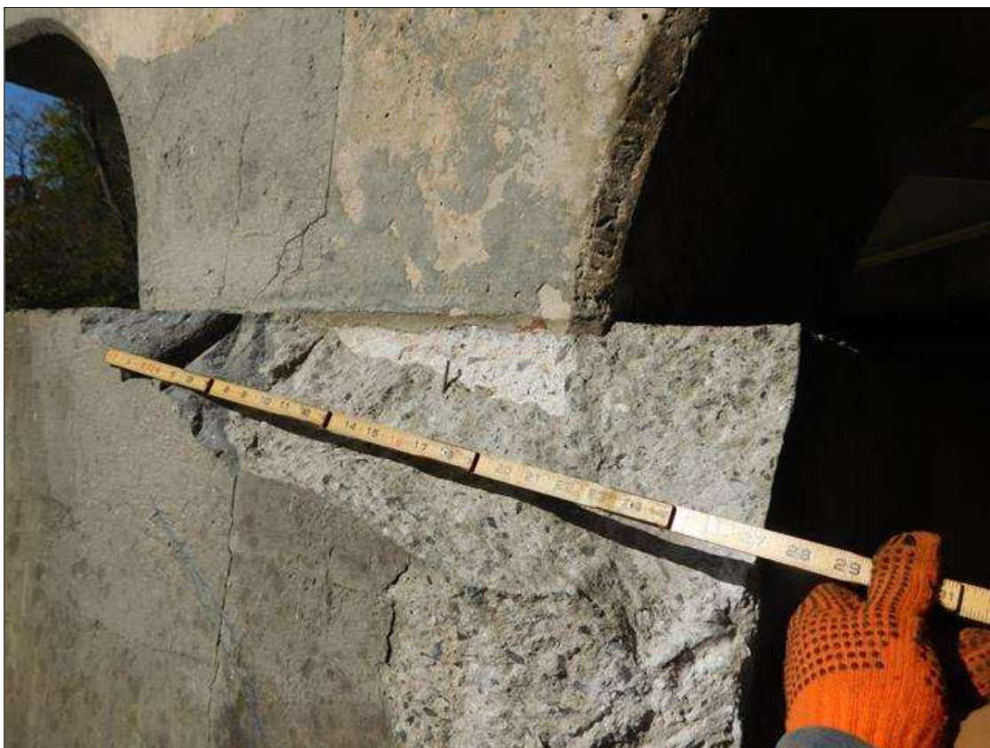
COLUMN 3 INT. BENT 1 SPALL 2'-10" HIGH X 2'-88" LONG X 7" DEEP AT THE TOP OF NEW SECTION (PAR)
