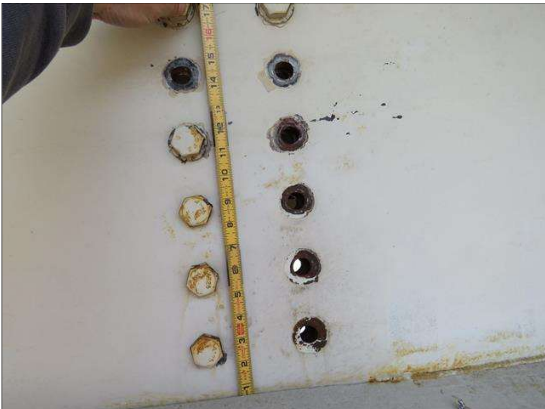
SPAN 3 DIAPHRAGM 2 BAY 1: 20 BOLTS WITH 6 MISSING ON BEAM 1, UP TO 1' HIGH CRACKING STRATING AT 1/32" WIDE AT TOP AND UP TO 1 1/8" AT BOTTOM OF DIAPHRAGM (PAR) .
