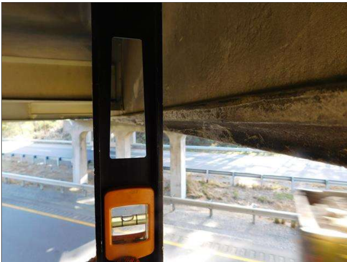
BEAM 2 SPAN 1 SWEPT EASTWARD 1 1/2" (PAR)
