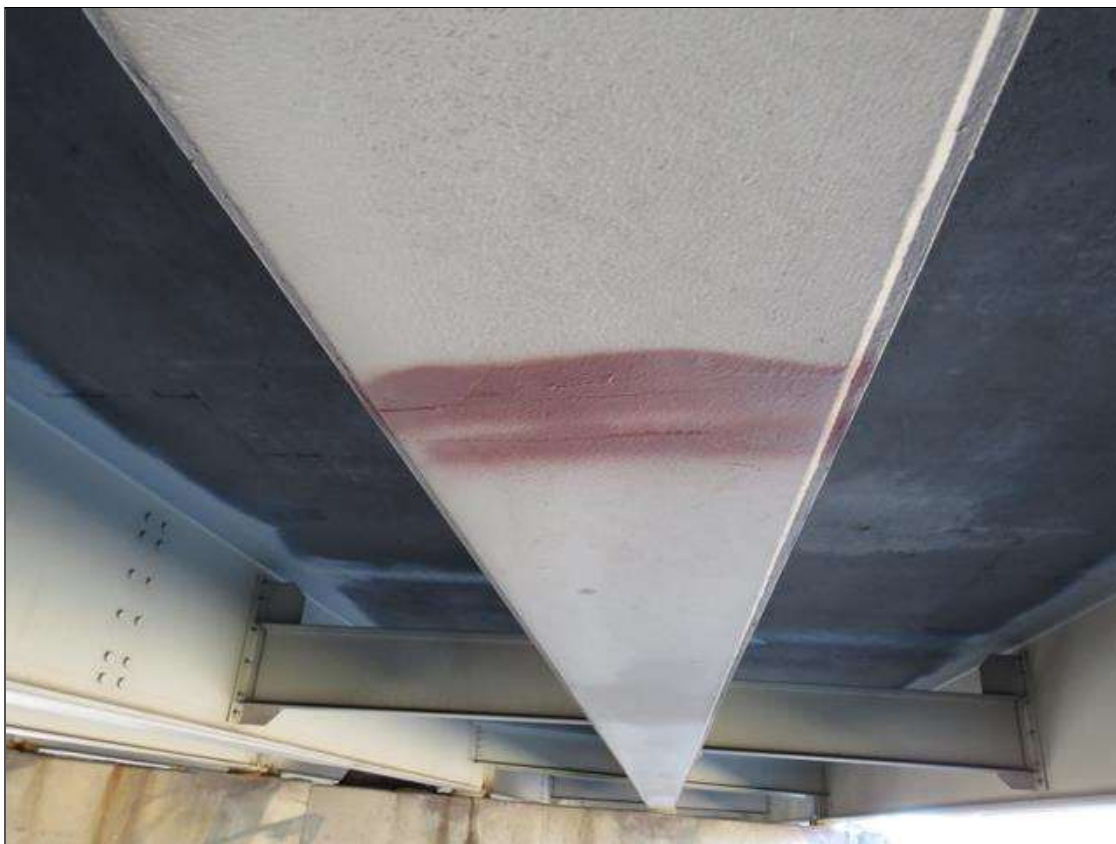
Span 3 Beam 2: SUPPLEMENTAL INSPECTION IMPACT DAMAGE 2021 :scattered scrapes
