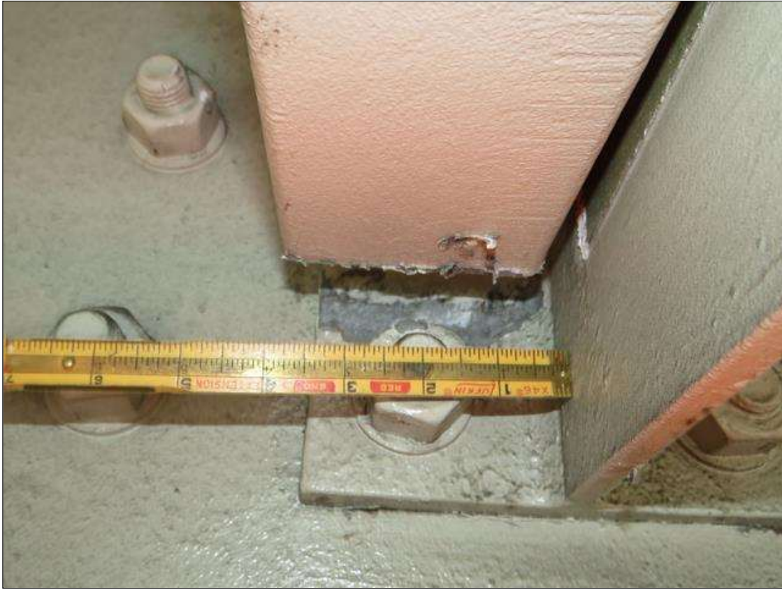
SPAN 2 BAY 1 BOTTOM LOWER BASE PLATE WELD BROKEN LOOSE FROM BEAM 1 DIAPHRAM 2 , 3 3/4" LONG X 1/16" DEEP AT 3" UP FROM BOTTOM OF PLATE .(PAR)
