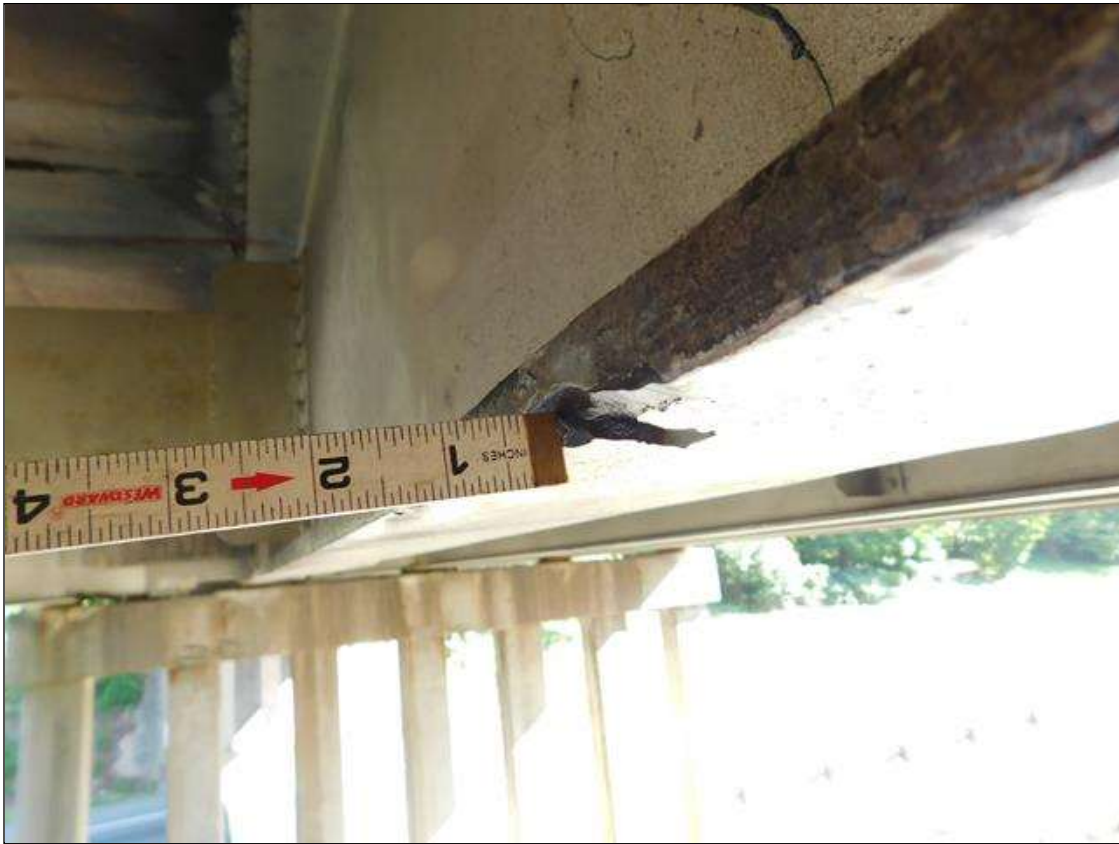
Span 2 Beam 2: SUPPLEMENTAL INSPECTION 2021: POINT OF IMPACT 8" LONG WITH A 1/2" DEEP GOUGE AT 18'-8" FROM INT. BENT 2 , WITH BEAM BEING SWEEP EASTWARD 1/2". SCATTERED SCRAPES ALONG THE BEAM (PAR) THERE IS A BENT UP SECTION ON THE WEST BOTTOM FLANGE 4" LONG X 1" HIGH AT 20' OUT FROM INT. BENT 1 (PAR)
