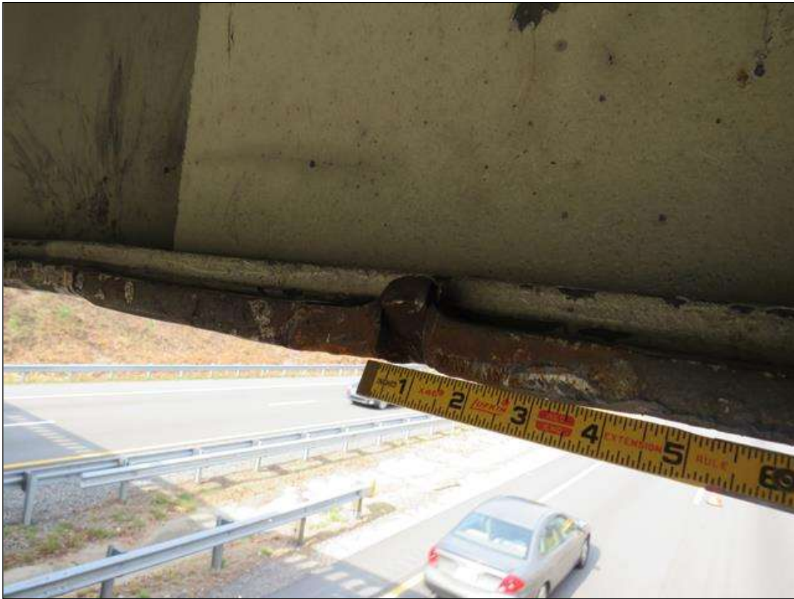
Span 3 Beam 1: SUPPLEMENTAL INSPECTION IMPACT DAMAGE 2022.: POINT OF IMPACT 9' LONG WITH SCATTERED 1" DEEP INDENTIONS THROUGH OUT BOTTOM FLANGE , AT 12'-9" OUT FROM INT. BENT 3 . BEAM 1 DEFLECTION 1/2" TO THE WEST. .,EAST SIDE OF BOTTOM FLANGE BENT UPWARD 1/2in. SCATTERED SCRAPES ALONG BOTTOM FLANGE. (PAR) . SCATTERED OLD SCRAPES AND INDENTIONS ALONG BOTTOM FLANGE .
