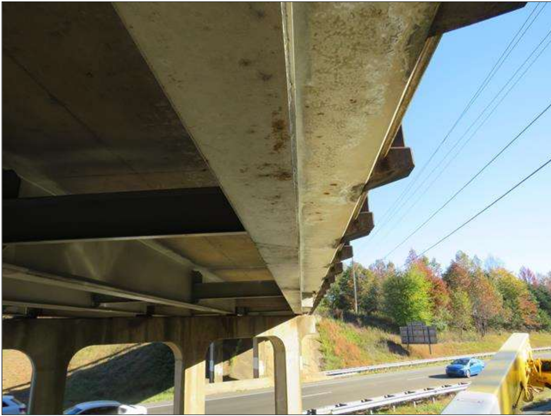
Span 2 Beam 4: SUPPLEMENTAL INSPECTION 2021: SCATTERED SCRAPS THROUGHOUT ON BOTTOM COVER PLATE
