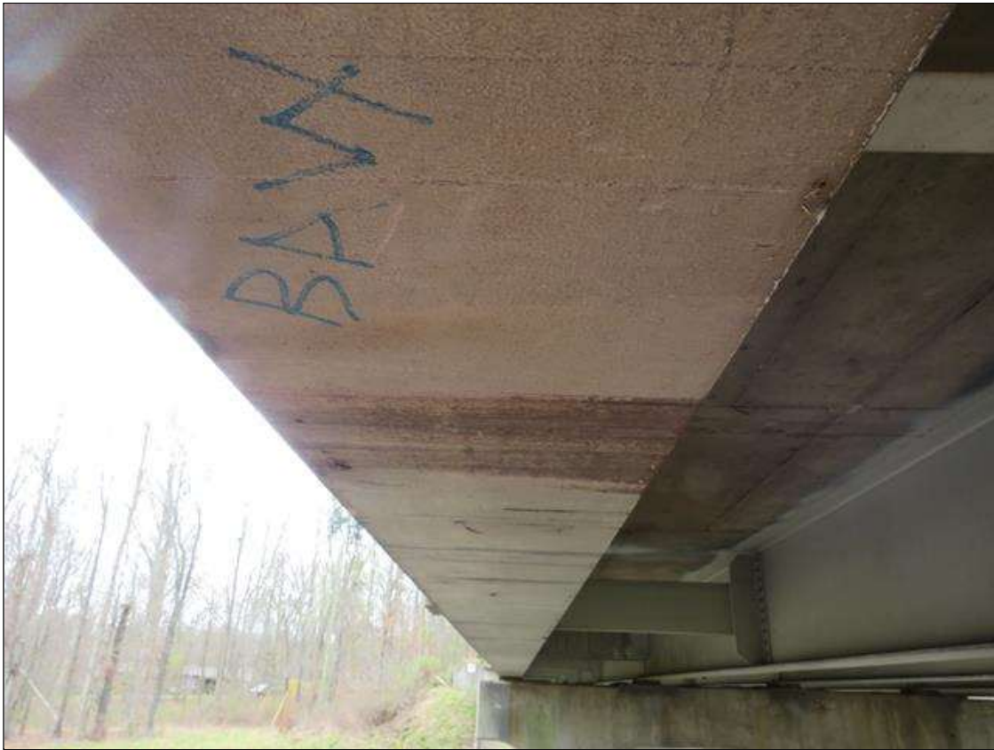
Span 3 Beam 5: beam 5 span 3 has scrapes on bottom flange
