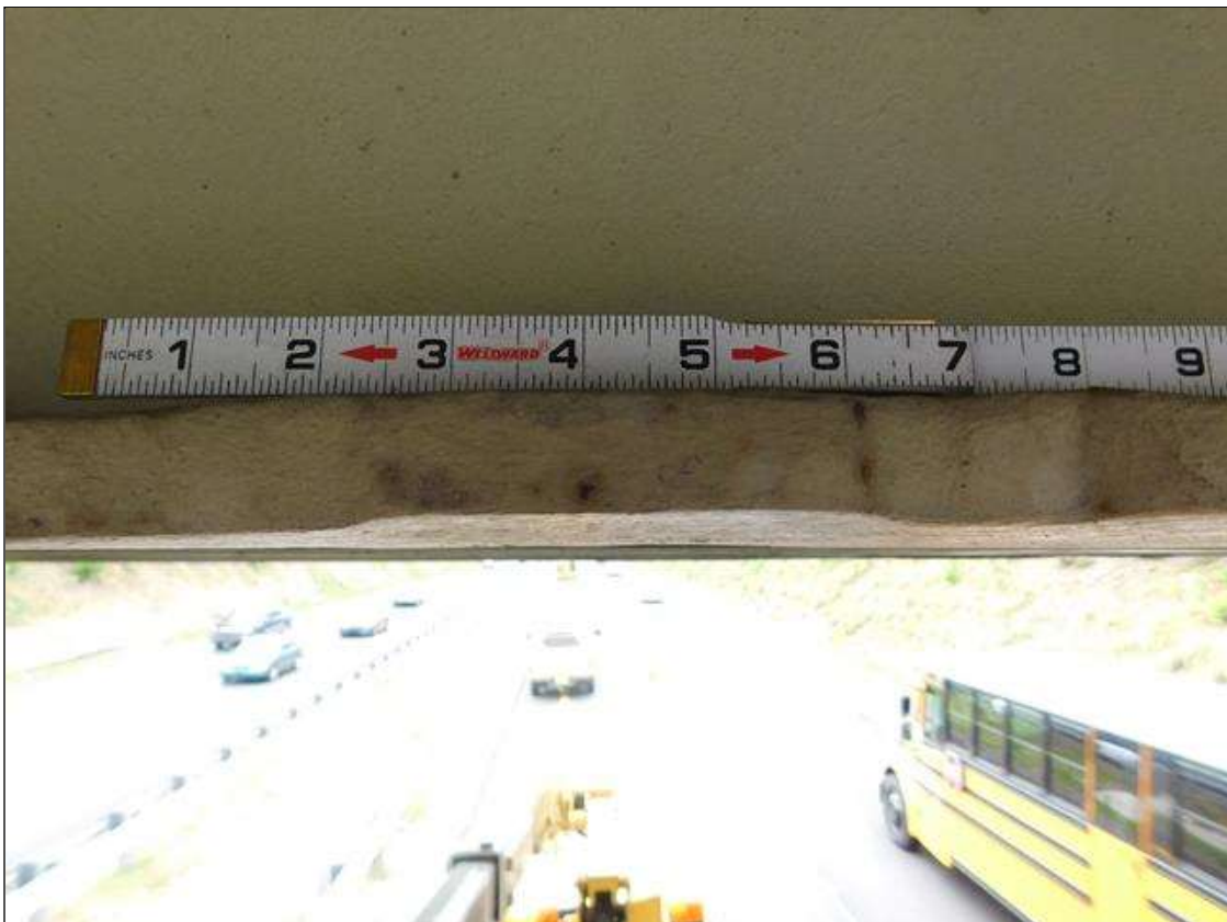
Span 3 Beam 3: TWO INDENTIONS IN BOTTOM FLANGE OF BEAM 3 SPAN 3. ONE 1/4" DEEP AND ONE 1/2" DEEP AT 15.583" FROM INTERIOR BENT 2 FOR A TOTAL LENGTH OF 1'
