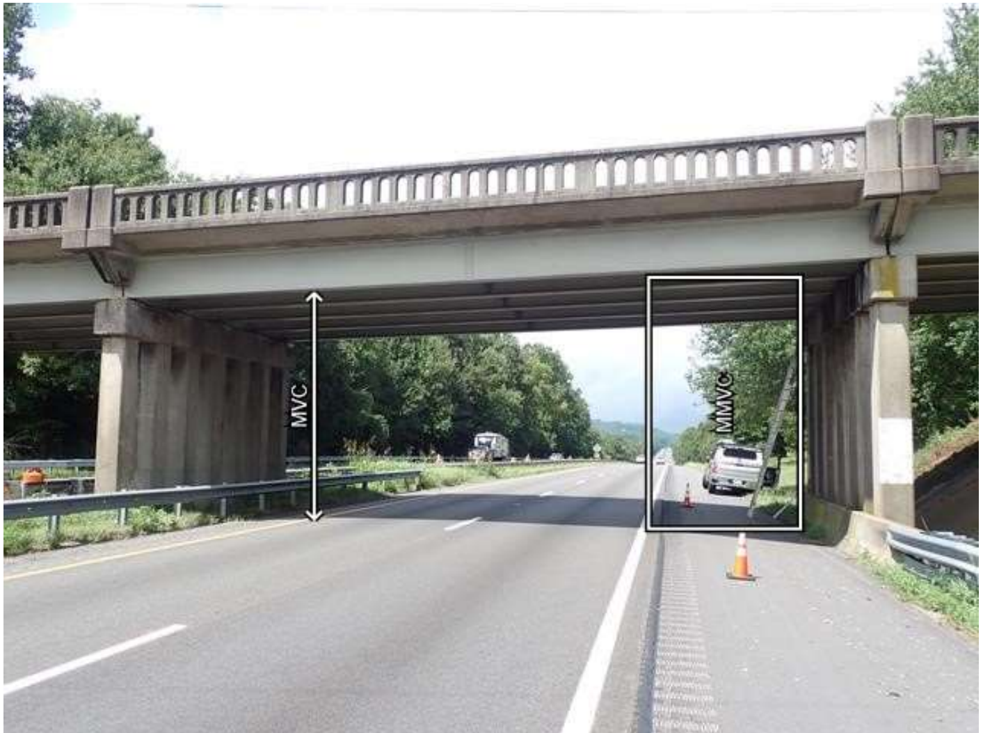
Span 3 vertical clearance looking West
