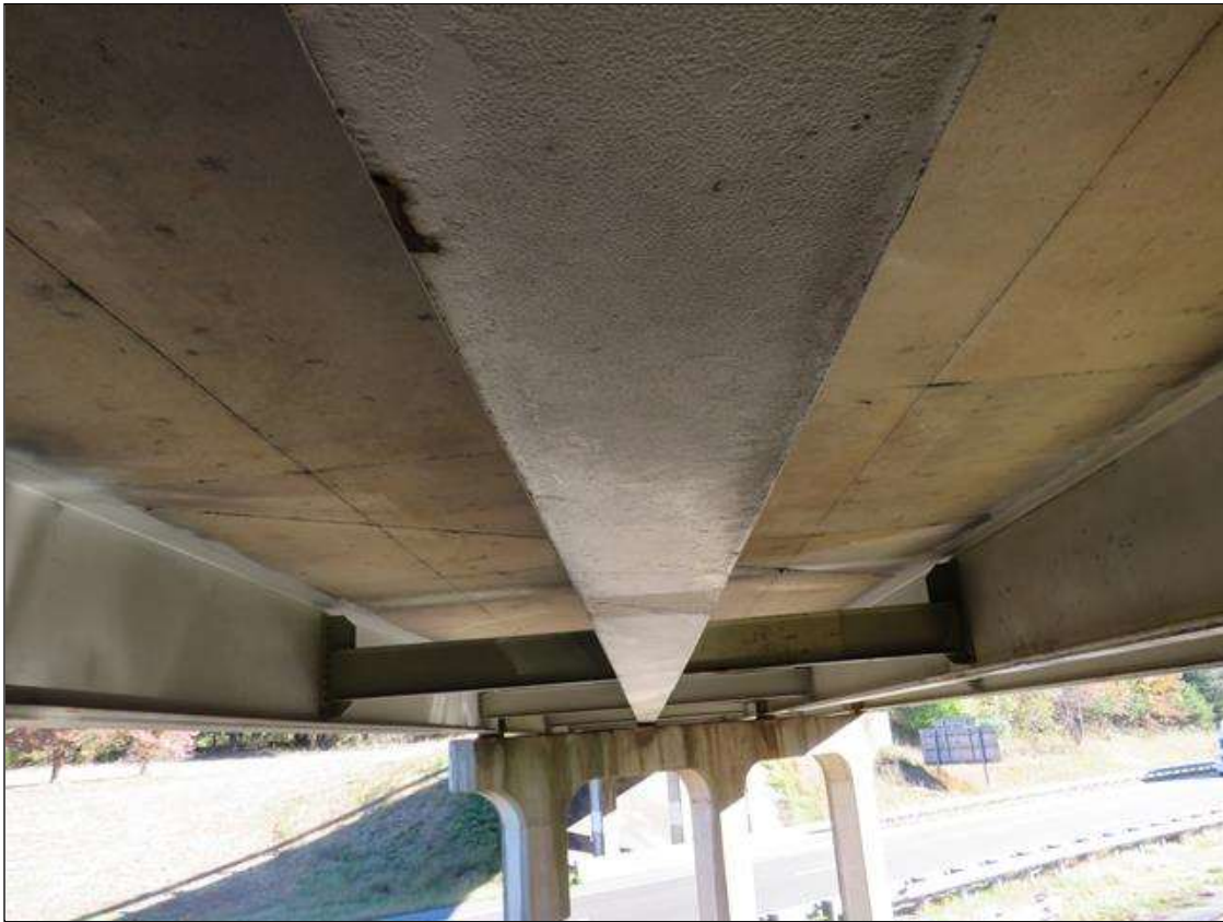
Span 2 Beam 2: SUPPLEMENTAL INSPECTION 2021: Point of impact on beam 2 West approach slab 27'-6" from face of bent 1. Gouges in flange cover plate 1/2" X 14" X 1/16" and a indentation in flange cover plate 6" X 1/32", a indentation in flange 1 1/2" X 1/16" all in the impact area.
