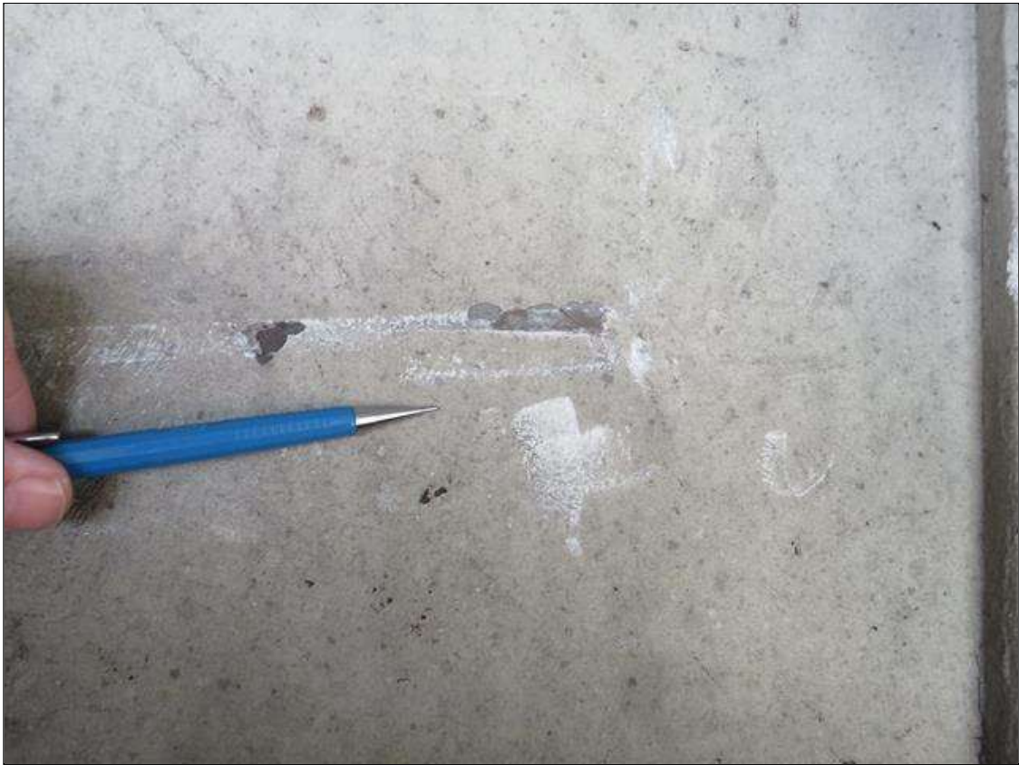
SCATTERED SCRAPES ALONG WEB BEAM 2 SPAN 3
