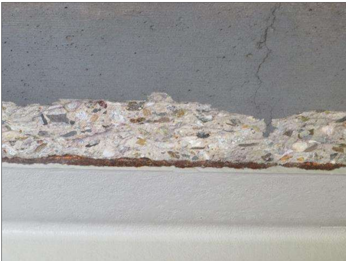
Span 3 Deck: SUPPLEMENTAL INSPECTION IMPACT DAMAGE 2022.: full length x up to 1/2in deep surface spalling, in underside of deck, along edges of beam 3.
