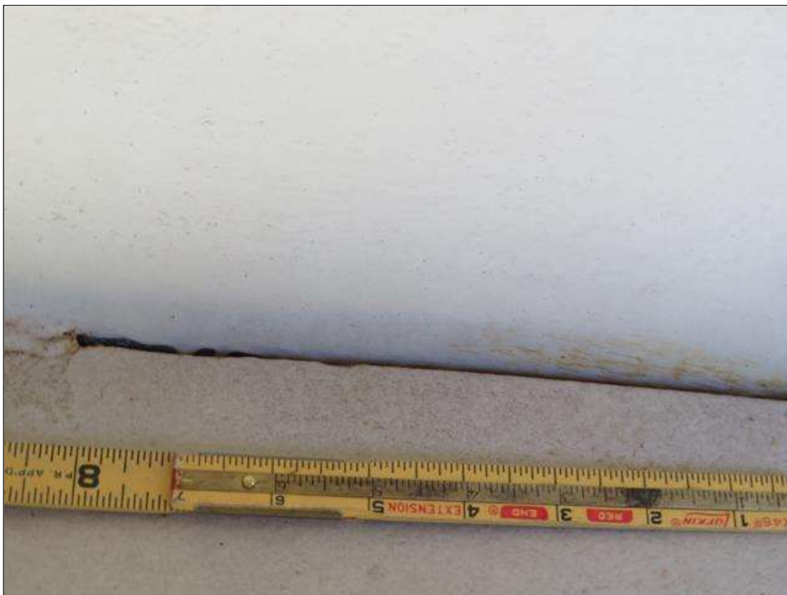
Span 3 Beam 1: SUPPLEMENTAL INSPECTION IMPACT DAMAGE 2022. Crack in weld of plate at TOP flange of beam 1 span 3 measured at 17ft from bent 3 for a length of 1ft
