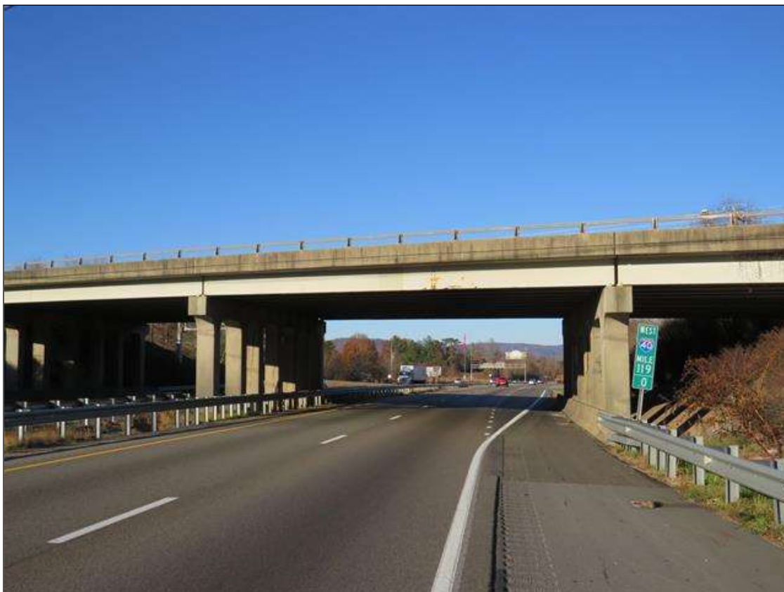
LOOKING WEST CLEARANCE
