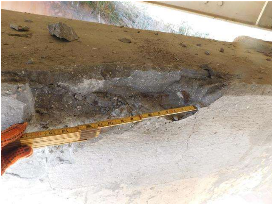
INT. BENT 1 CAP SPALL 26" LONG X 9" HIGH X 5" DEEP AT 8'-6" FROM EAST END BAY 3 WITH 1 REINFORCING BAR EXPOSED (PAR)
