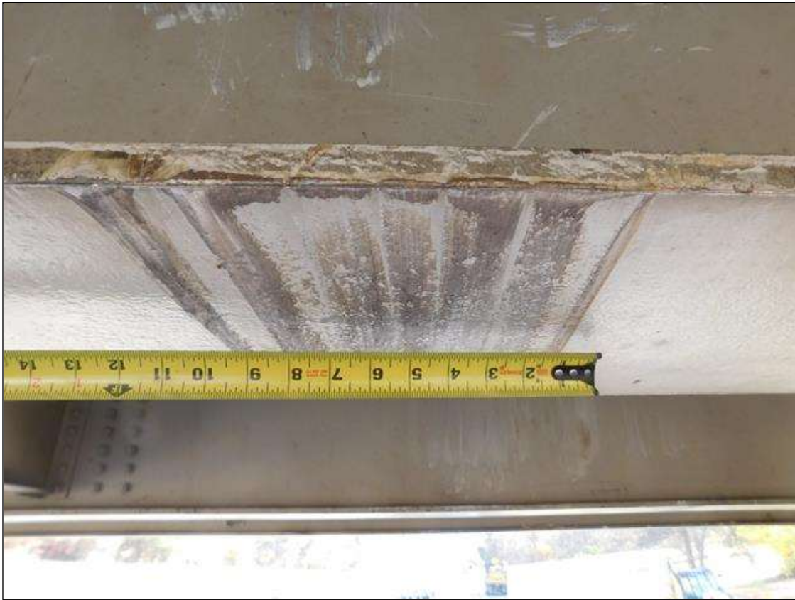
Span 2 Beam 3: SCRAPES TO BOTTOM FLANGE AT 20'9" FROM INT. BENT 1
