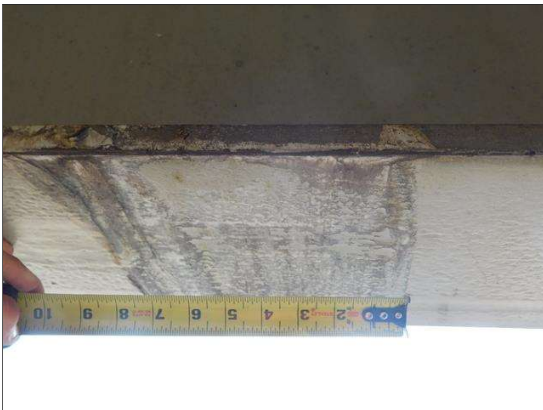
Span 2 Beam 5: SCATTERED SCRAPES TO BOTTOM FLANGE
