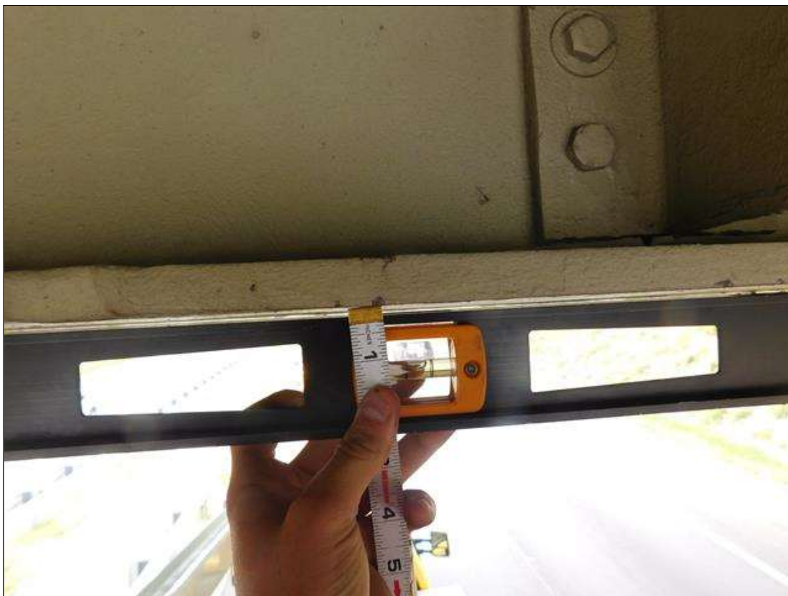
Span 3 Beam 3: BEAM 3 SPAN 3 DEFLECTED UPWARD 1/4" FOR A LENGTH OF 3' AT 15' FROM INTERIOR BENT 2
