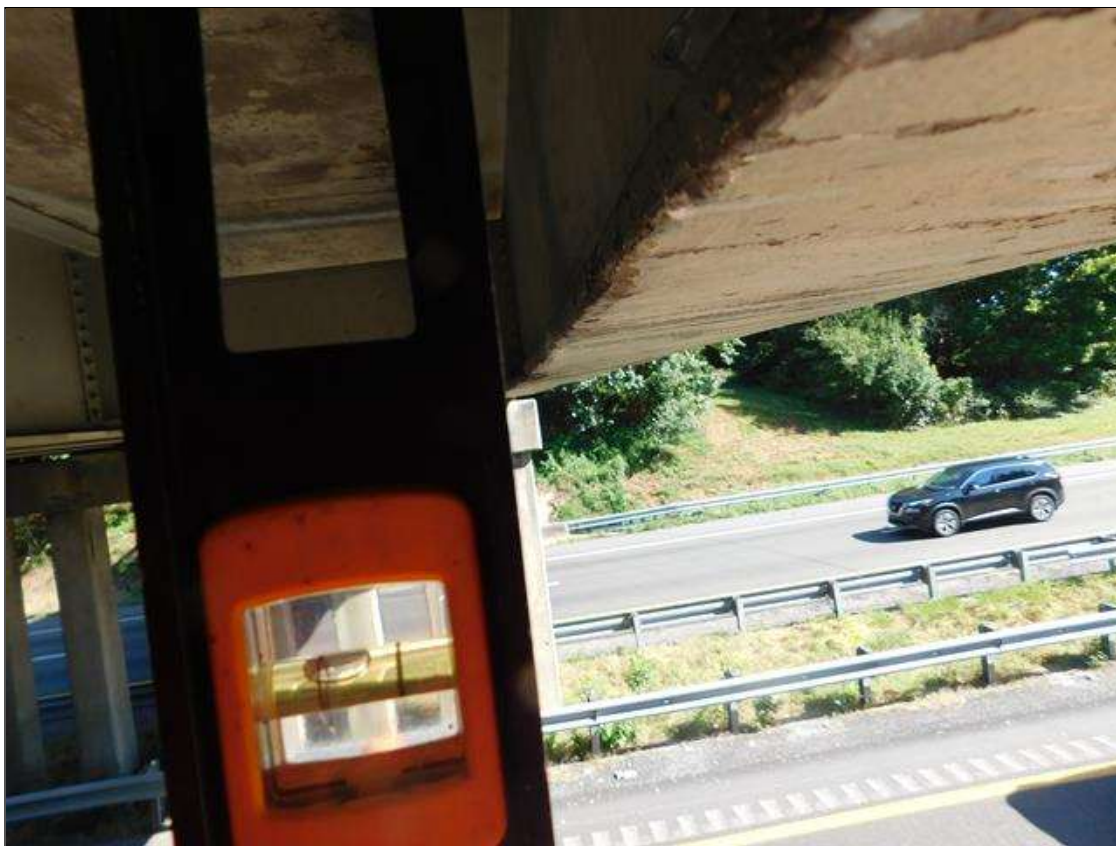
Span 2 Beam 5: 2021 SUPPLEMENTAL INSPECTION 2021 : BEAM 5 SPAN 2 POINT OF IMPACT 10" LONG X 1" HIGH AT 14'10" OUT FROM INT. BENT 2 , WITH THE BEAM BEING SWEEPED EAST WARD UP TO 3" .SCATTERD SCRAPES ALONG THE BOTTOM FLANGE . PREVIOUS IMPACT DAMAGE AS NOTED IN THE ADDITIONAL COMMENTS SECTION. (PAR)
