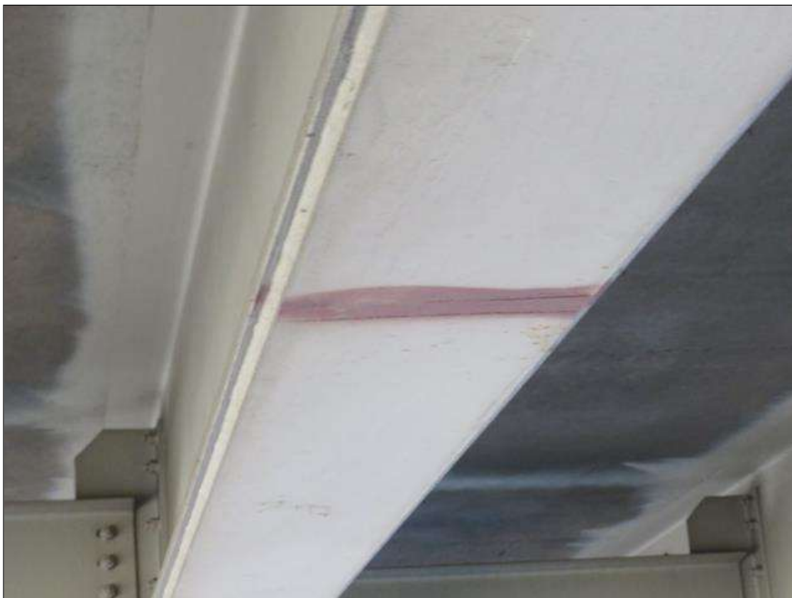
Span 3 Beam 3: SUPPLEMENTAL INSPECTION IMPACT DAMAGE 2021 :scattered scrapes
