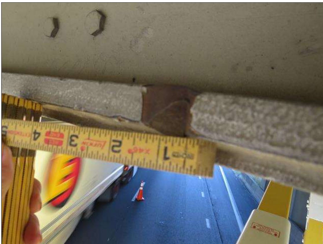
Span 3 Beam 9: SUPPLEMENTAL INSPECTION IMPACT DAMAGE 2021: 1 indentation 1" long x 1/4" deep at 18'-7" from int. bent 3
