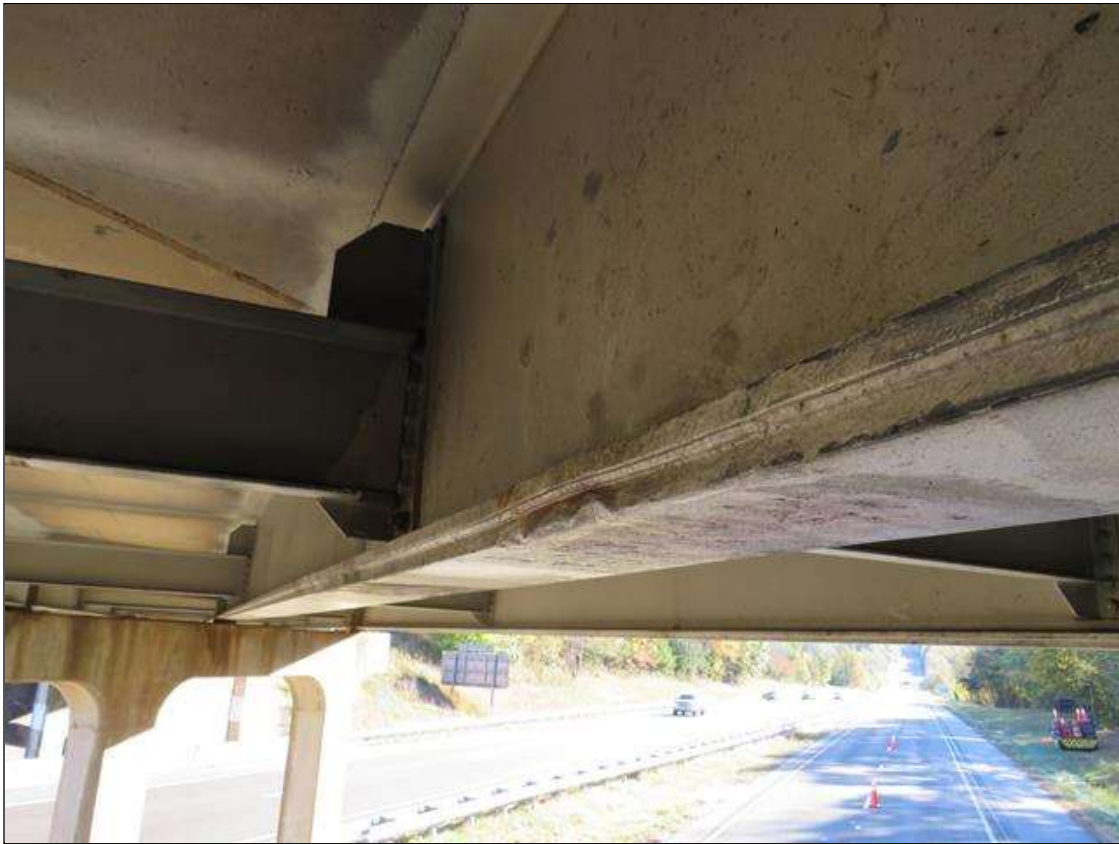
Span 2 Beam 3: SUPPLEMENTAL INSPECTION 2021: Point of impact on beam 3 West approach slab 26'-1" from face of bent 1. Beam 1 is out of plumb 2 1/2" +/- in the direction of traffic and a indentation in cover plate 3" X 1/2" and a 2" X 1/2" in the impact area.
