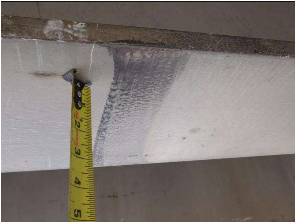
Span 2 Beam 4: SCATTERED SCRAPES TO BOTTOM FLANGE
