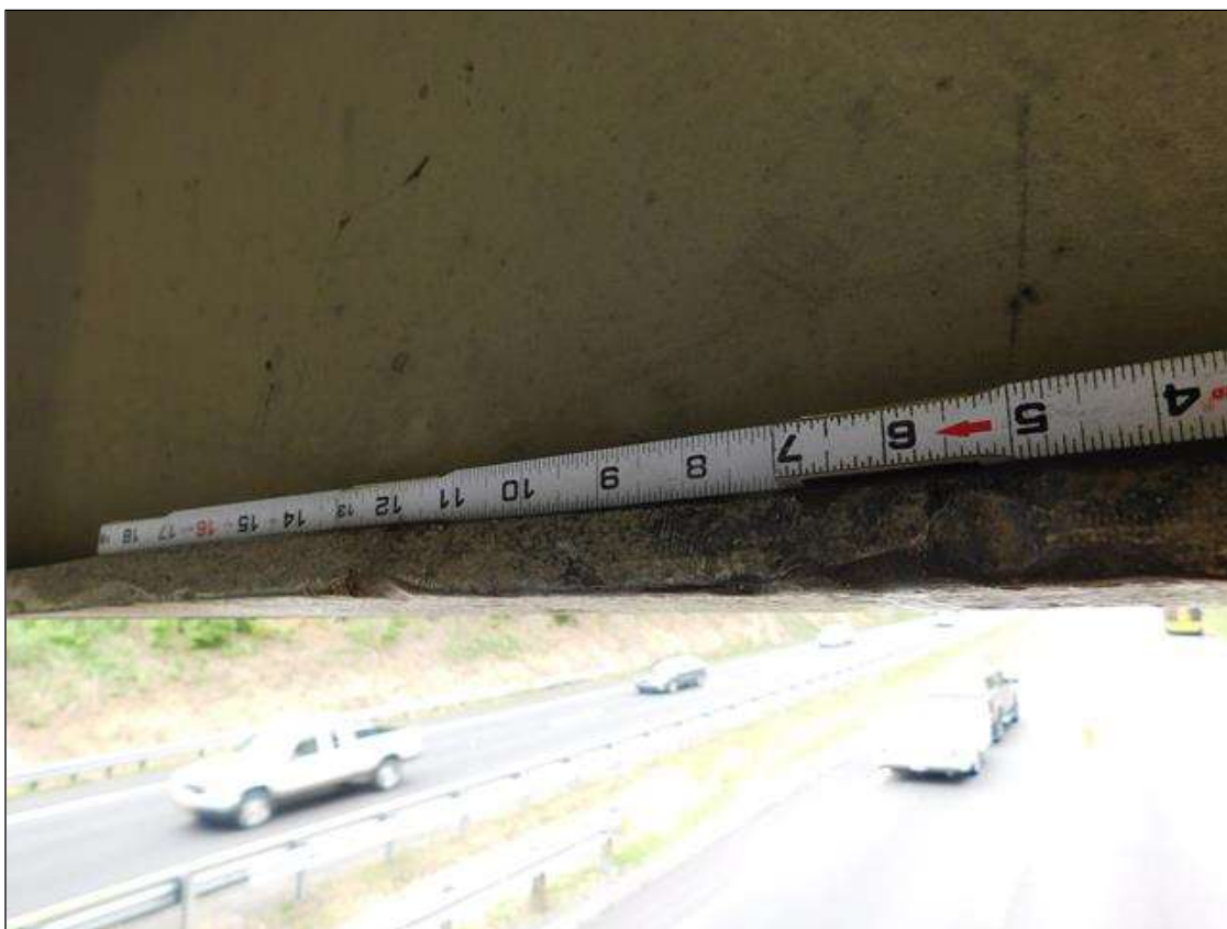
Span 3 Beam 2: MINOR INDENTIONS IN BEAM 2 SPAN 3 STARTING AT 18.167' FROM INTERIOR BENT 3 FOR A TOTAL LENGTH OF 2'
