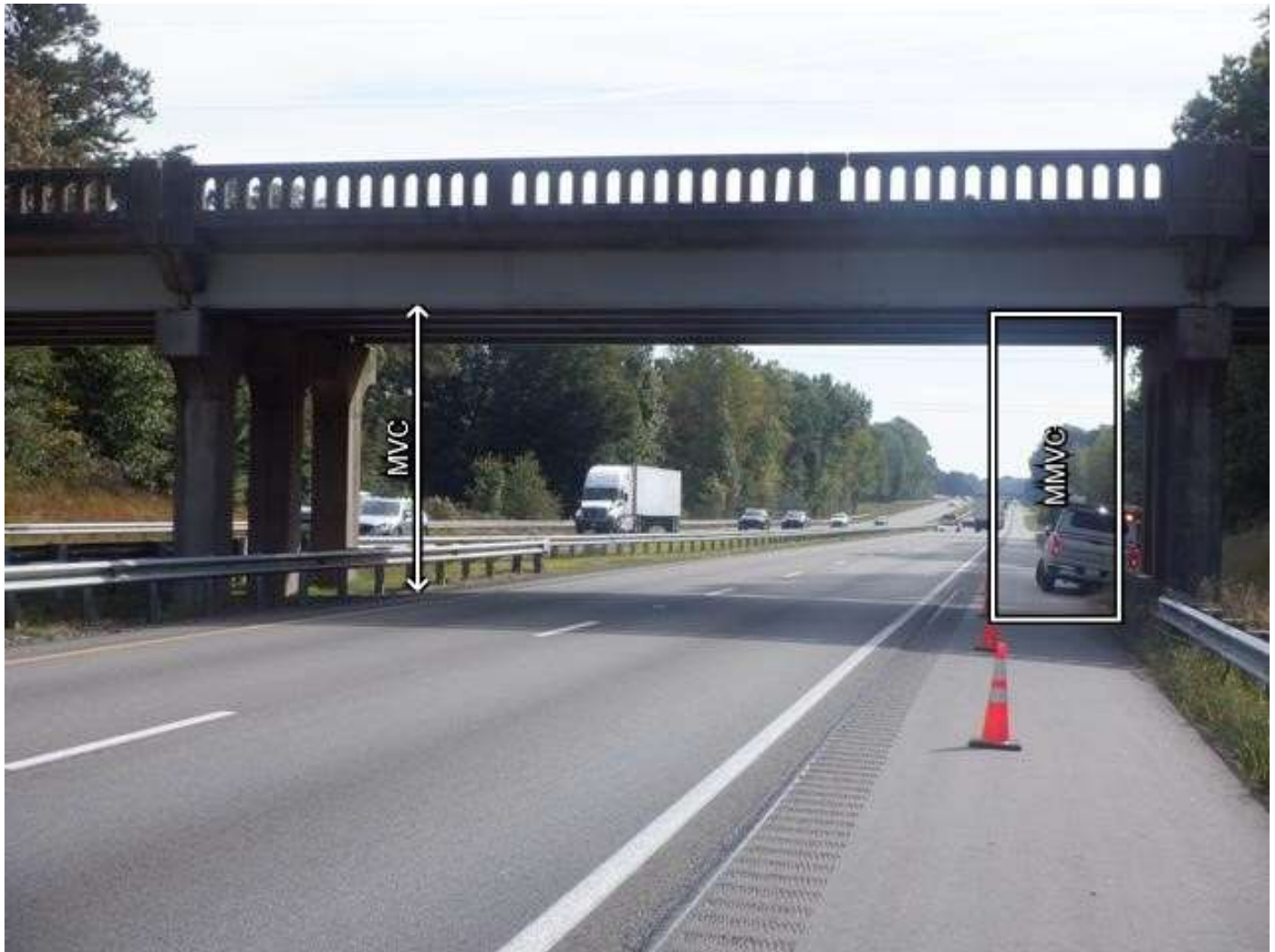
vertical clearance looking East [span 2]
