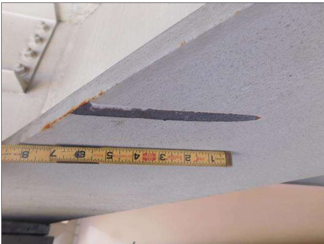
BEAM 2 SPAN 1 SCATTERED SCRAPES BOTTOM FLANGE OF BEAM 2
