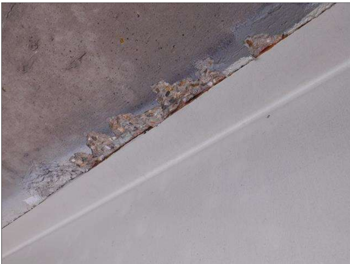
Span 3 Beam 3: SPALL AT EAST SIDE OF TOP FLANGE OF BEAM 3 SPAN 3. 3' LONG AT 12' FROM INTERIOR BENT 2
