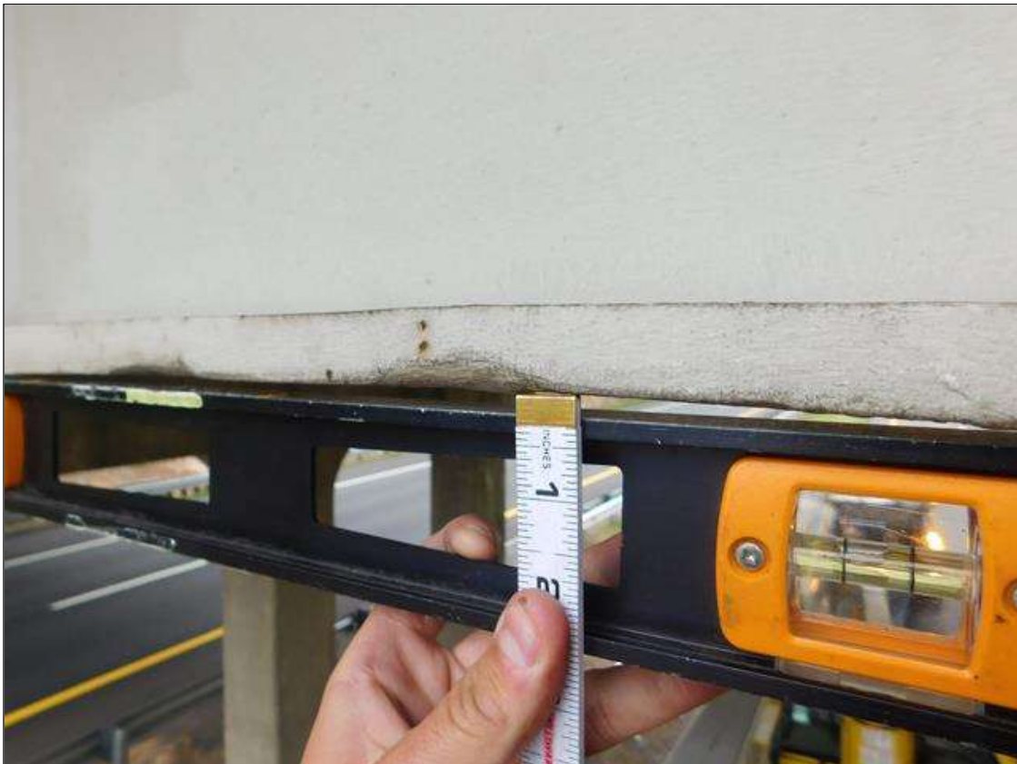
Span 3 Beam 5: BEAM 5 SPAN 3 IS DEFLECTED UPWARD 1/4" AT 16.417' FROM INTERIOR BENT 2 FOR A LENGTH OF 3'
