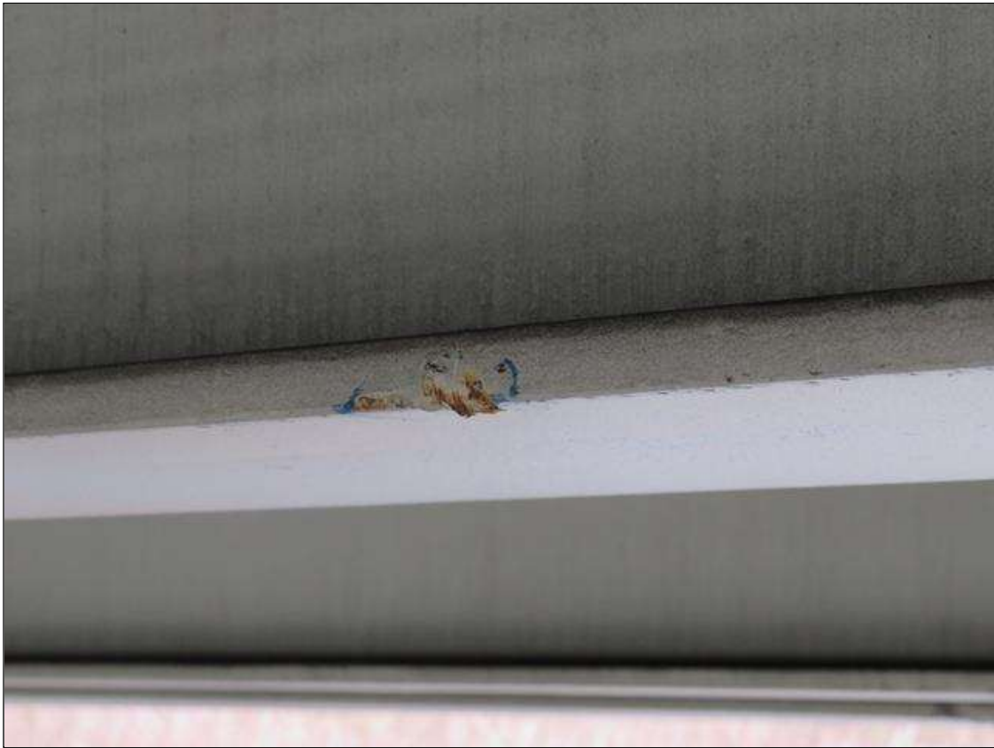
Span 2 Beam 2: 2022 OLD INDENTIONS BEAM 4
