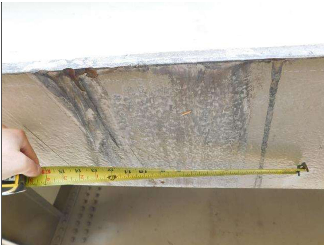
SPAN 2 BEAM 1: SCATTERED SCRAPES TO BOTTOM FLANGE
