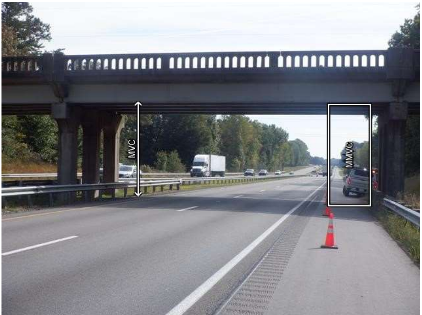
vertical clearance looking East [span 2]
