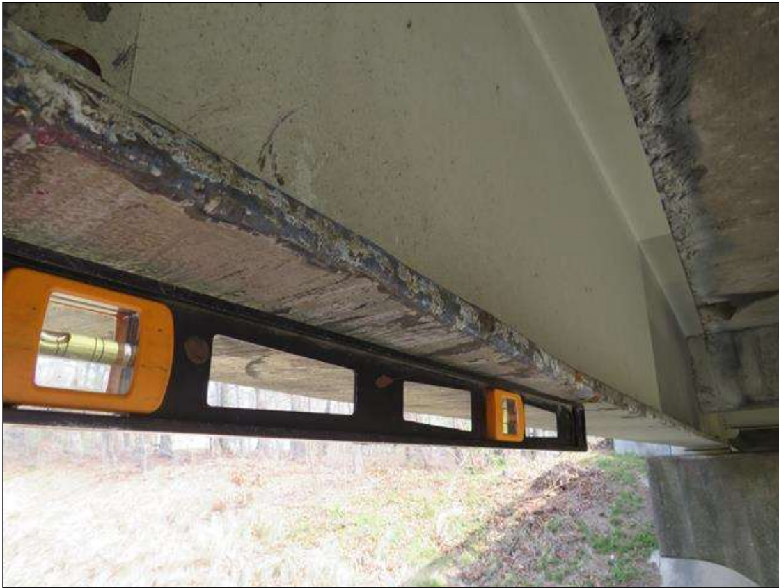
Span 3 Beam 1: SUPPLEMENTAL INSPECTION IMPACT DAMAGE 2022.: POINT OF IMPACT 9' LONG WITH SCATTERD 1" DEEP INDENTIONS THROUGH OUT BOTTOM FLANGE , AT 12'-9" OUT FROM INT. BENT 3 . BEAM 1 DEFLECTION 1/2" TO THE WEST. .,EAST SIDE OF BOTTOM FLANGE BENT UPWARD 1/2in. SCATTERED SCRAPES ALONG BOTTOM FLANGE. (PAR) . SCATTERED OLD SCRAPES AND INDENTIONS ALONG BOTTOM FLANGE .
