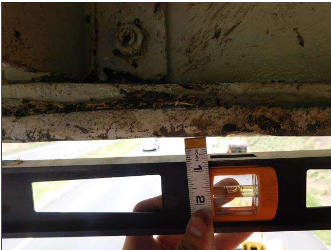
Span 3 Beam 1: BEAM 1 SPAN 3 IS DEFLECTED UPWARD 1" STARTING AT 14.583' FROM INTERIOR BENT 3 FOR A TOTAL LENGTH OF 6'
