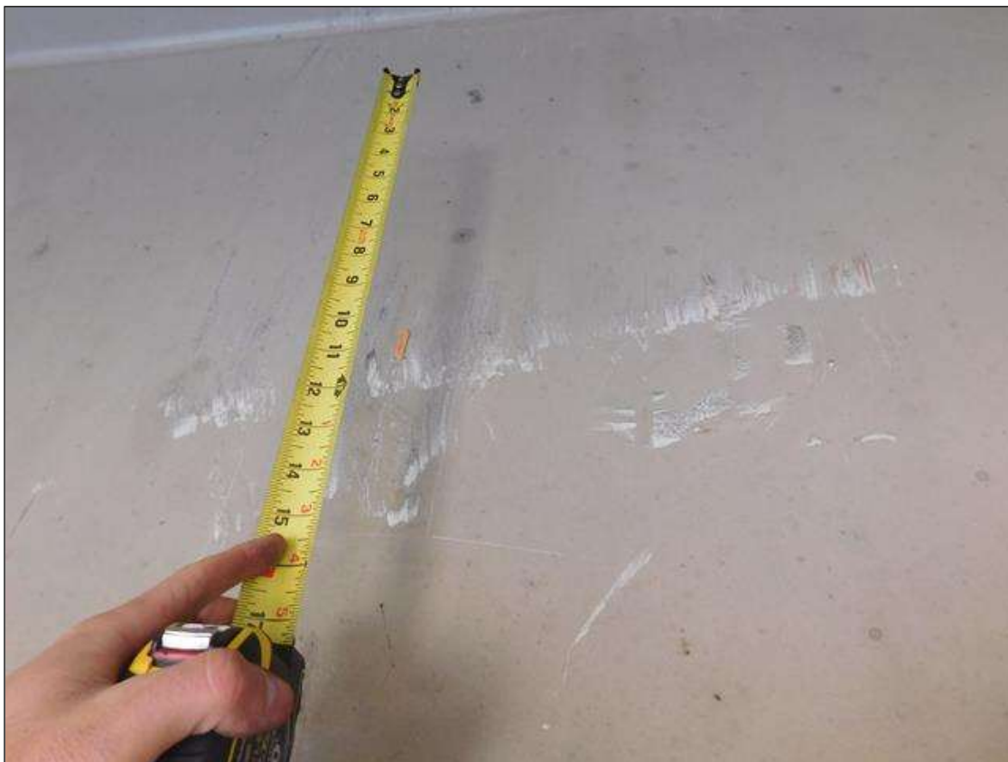
Span 2 Beam 3: SCATTERED SCRAPES TO LEFT SIDE OF WEB THROUGHOUT BEAM 3 SPAN 2
