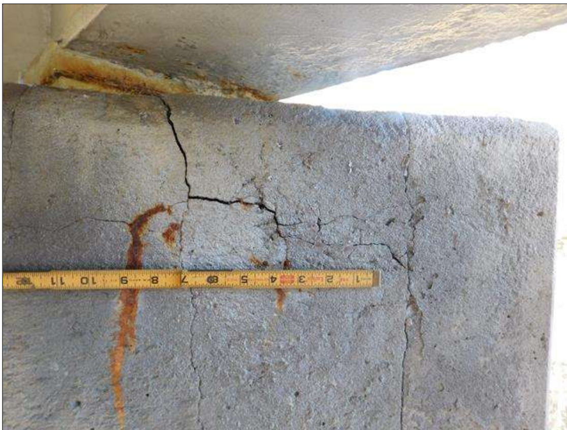
SCATTERED CRACKING IN CAP AT INT BENT 1 BENEATH BEAM 1 SPAN 2
