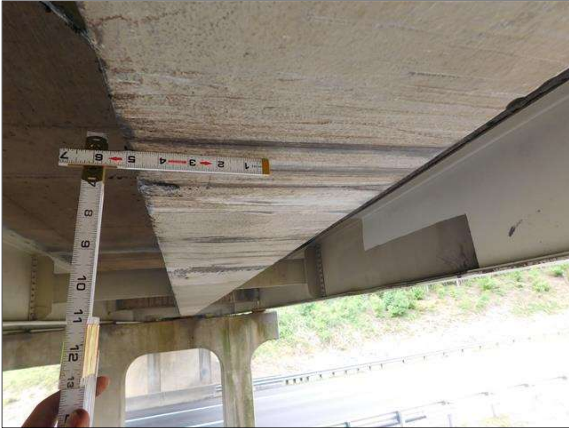
Span 3 Beam 2: DAMAGE TO BEAM 2 SPAN 3 STARTING AT 15.333' FROM INTERIOR BENT 3 FOR A TOTAL LENGTH OF 5', WITH SCRAPES THROUGHOUT BOTTOM FLANGE. POINT OF IMPACT MEASURED AT 16.917' FROM INTERIOR BENT 3
