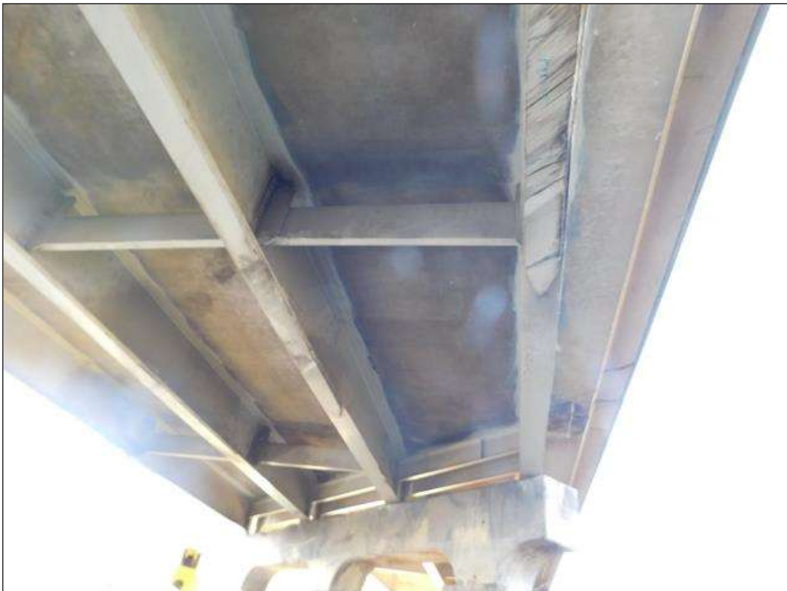
OVERVIEW OF DAMAGE SPAN 2 INT. BENT1
