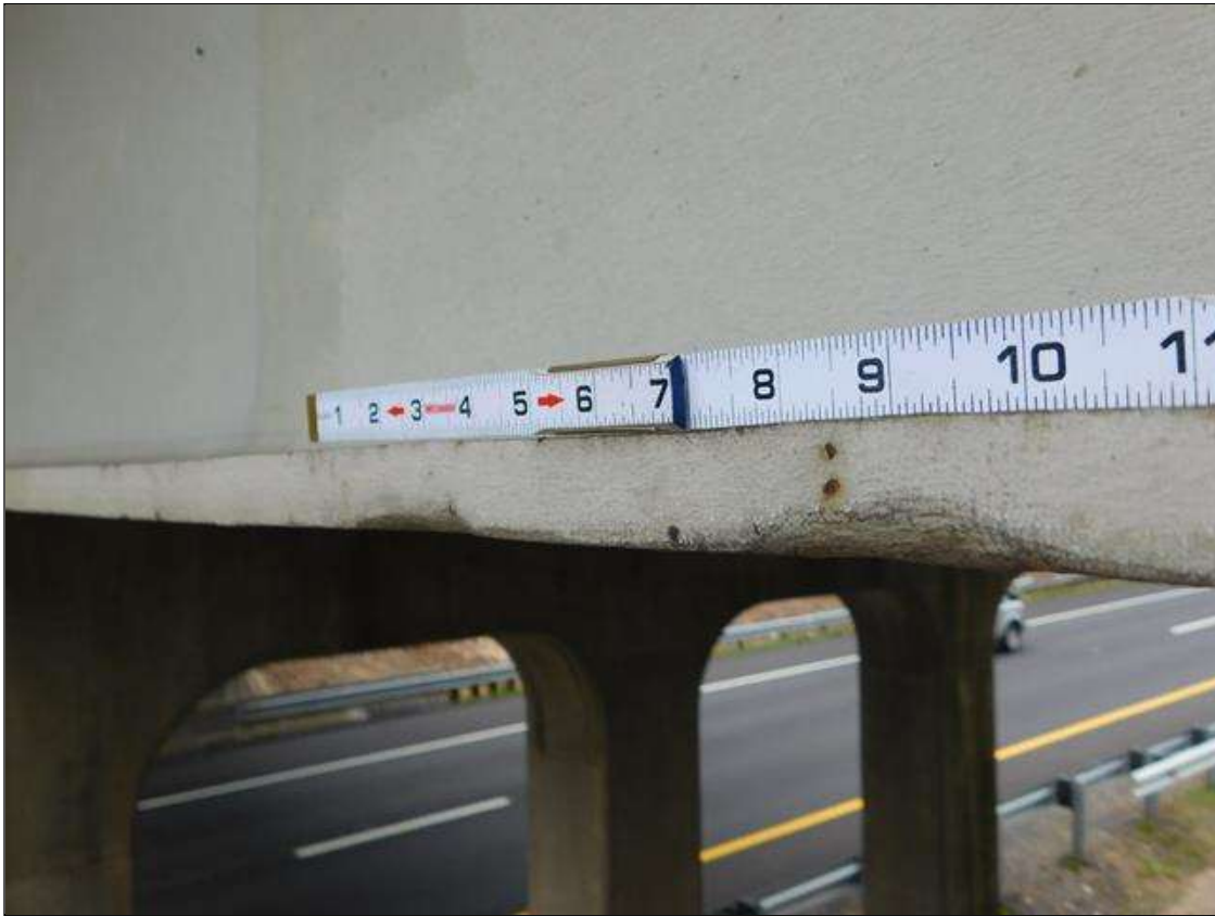
Span 3 Beam 5: TWO 1/4" DEEP INDENTIONS IN BOTTOM FLANGE OF BEAM 5 SPAN 3 AT 16.5' FROM INTERIOR BENT 2 FOR A LENGTH OF 1'
