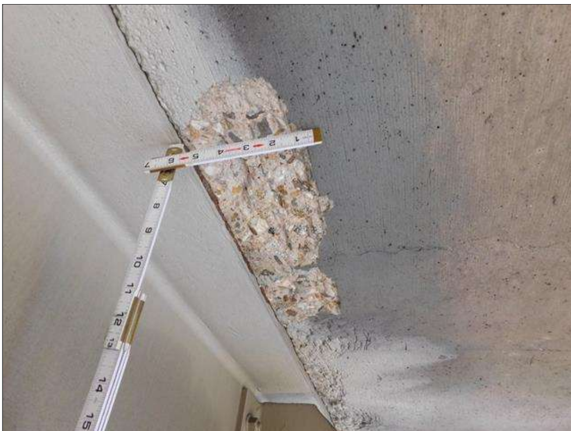
Span 3 Beam 2: SPALL AT TOP FLANGE OF WEST SIDE OF BEAM 2 SPAN 3. 17" LONG BY 6" WIDE BY 1/4" DEEF MEASURED AT 15.417' FROM INTERIOR BENT 3
