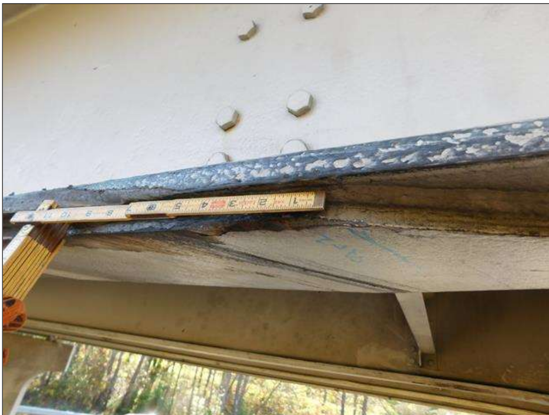
BEAM 1 SPAN 2 POINT OF IMPACT 2' LONG X WITH 1/16" INDENTIONS AT 14'-6" OUT FROM INT. BENT 1(PAR)
