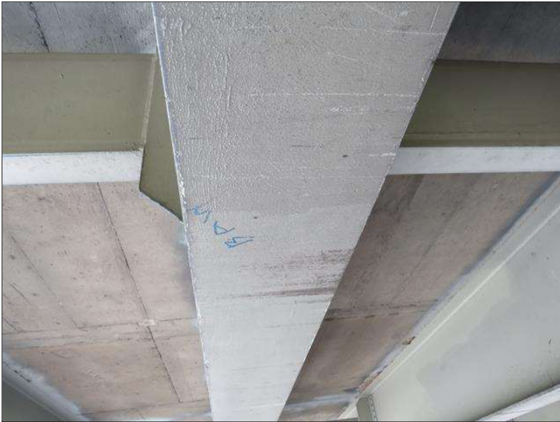
Span 3 Beam 4: SUPPLEMENTAL INSPECTION IMPACT DAMAGE 2022.: Beam 4 Span 3 has scrapes to bottom flange at 16.75ft from bent 3 for a total length of 1ft
