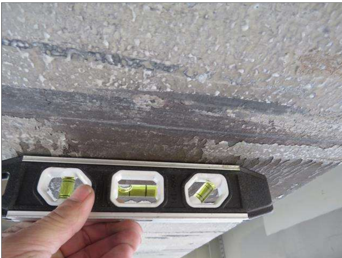
Span 3 Beam 2: SUPPLEMENTAL INSPECTION IMPACT DAMAGE 2022.: beam 2 span 3 deflected upward 1/2in at 19.5in from bent 2 for a length of 4ft, with scrapes on bottom flange
