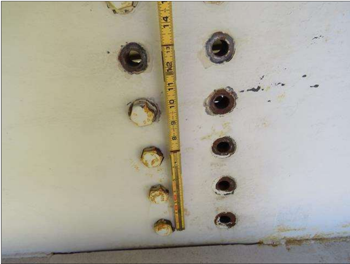
6 DIAPHRAGM BOLTS MISSING BEAM 1
