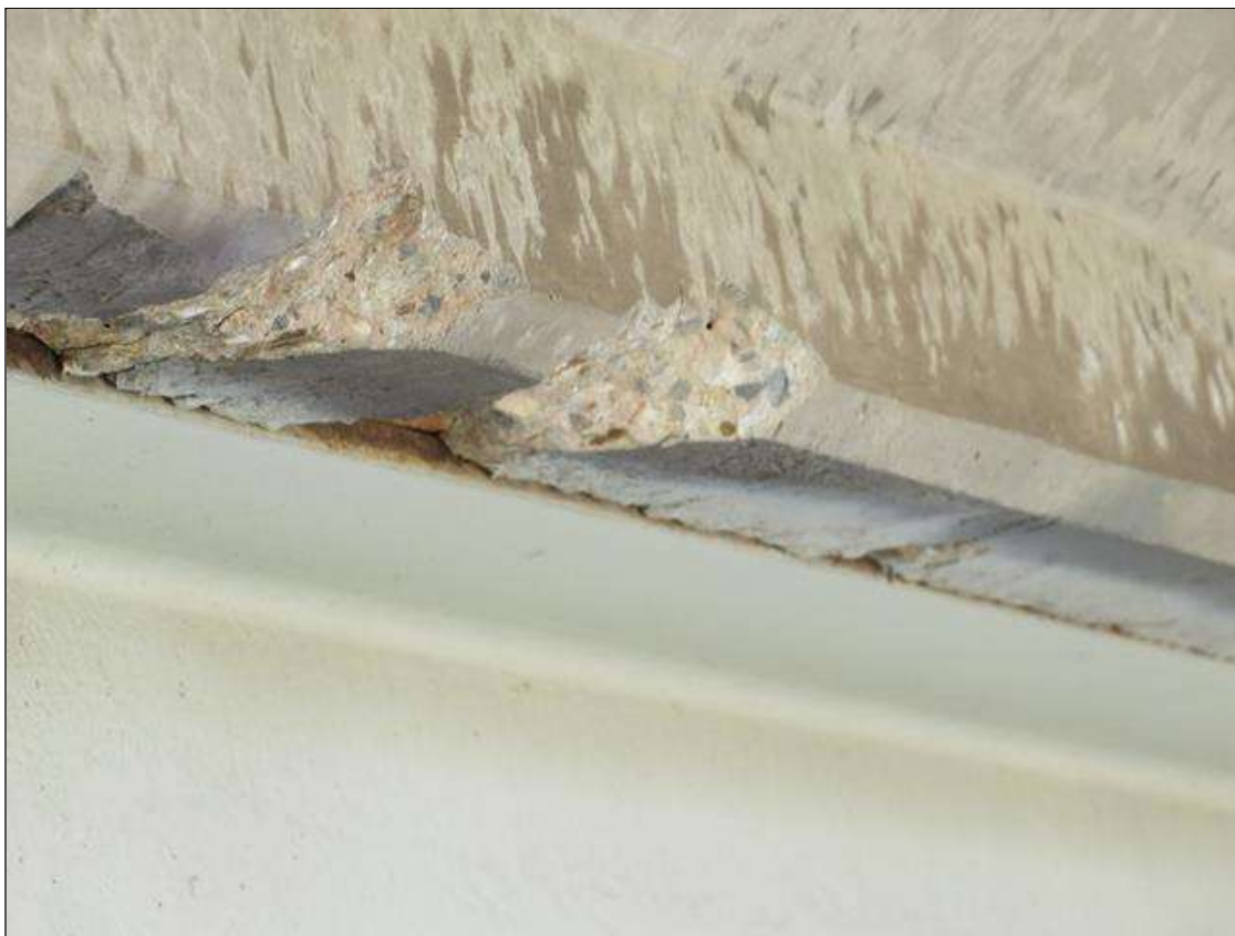
Span 3 Deck: SUPPLEMENTAL INSPECTION IMPACT DAMAGE 2022. spalling up to 12" WIDE X 1" deep, full length, underside of deck along both sides of beam 1.
