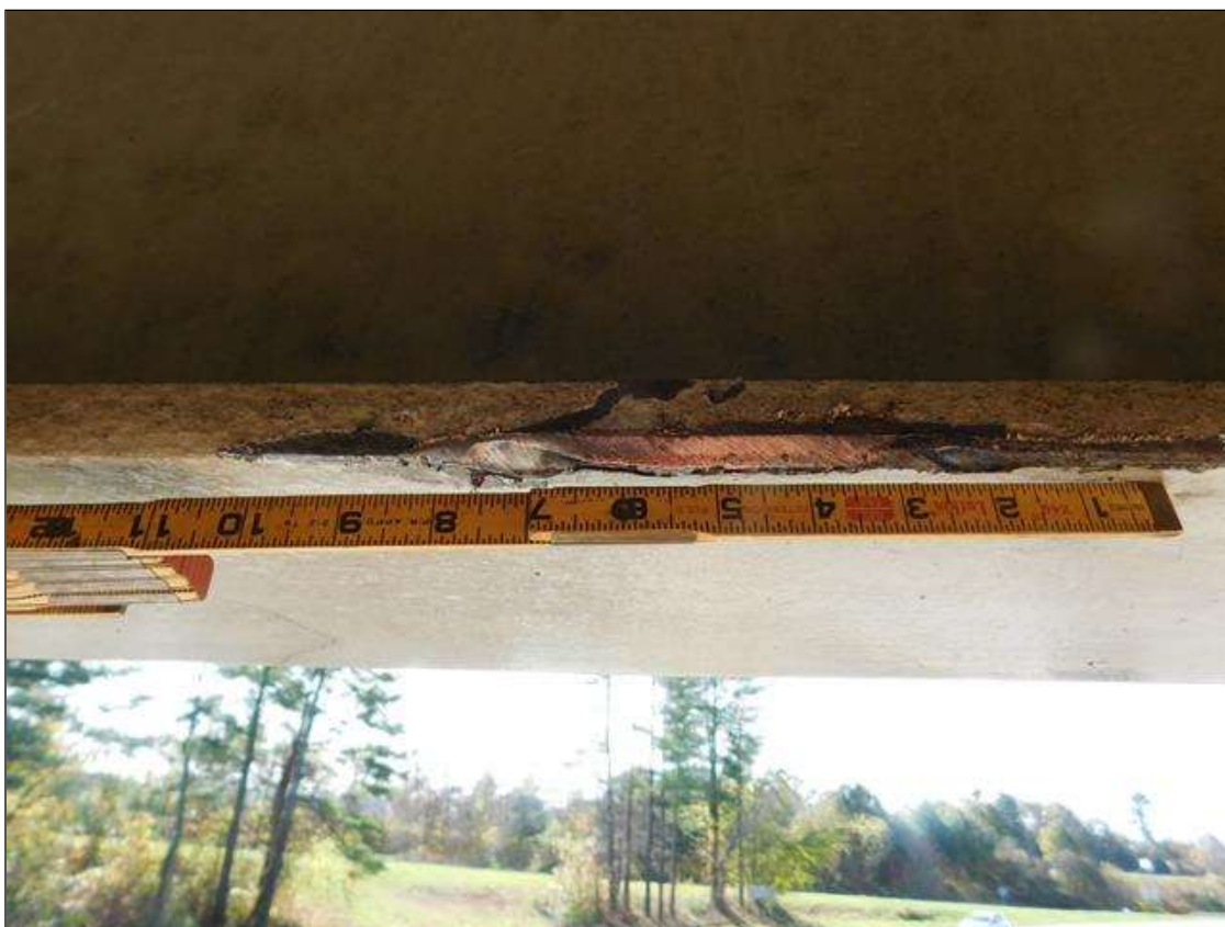
BEAM 4 SPAN 1 SCRAPE 11" LONG X 1/16" DEEP AT 9'-3" OUT FROM INT. BENT 1
