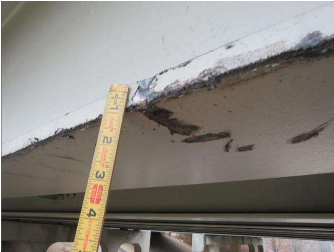
Span 2 Beam 1: SUPPLEMENTAL INSPECTION IMPACT DAMAGE 2022: SPAN 2 BEAM 1 ,BEAM SWEEP SOUTHWARD UP TO 3" X 25' LONG . (POI )8' OUT FROM INT. BENT 1 WITH A LENGTH OF 10' . 1 INDENTION 1/8" DEEP X 3" LONG AT 10' OUT FROM INT. BENT 1. WITH 2 OTHER INDENTIONS AT 16'-7" OUT FROM INT. BENT 1 , 22" LONG 1/4" WIDE X 1/16" DEEP AND 1/2" LONG X 1/4" DEEP . BOTTOM FLANGE OF BEAM BOWED UPWARD 1/2" . ANCHOR BOLT 1 LEFT SIDE BEAM 1 BENT WESTWARD . SCATTERED SCRAPES BEAM 1 BOTTOM FLANGE . (PAR)
