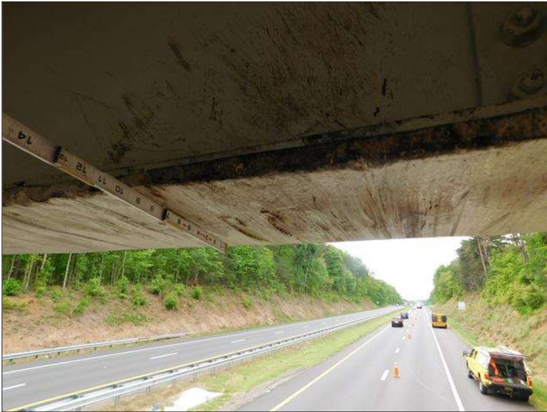
Span 3 Beam 1: DAMAGE TO BEAM 1 SPAN 3 STARTING AT 13.5' FROM INTERIOR BENT 3 FOR A TOTAL LENGTH OF 10'. POINT OF IMPACT MEASURED AT 17.417' FROM INTERIOR BENT 3, WITH SCATTERED SCRAPES AND INDENTIONS THROUGHOUT.
