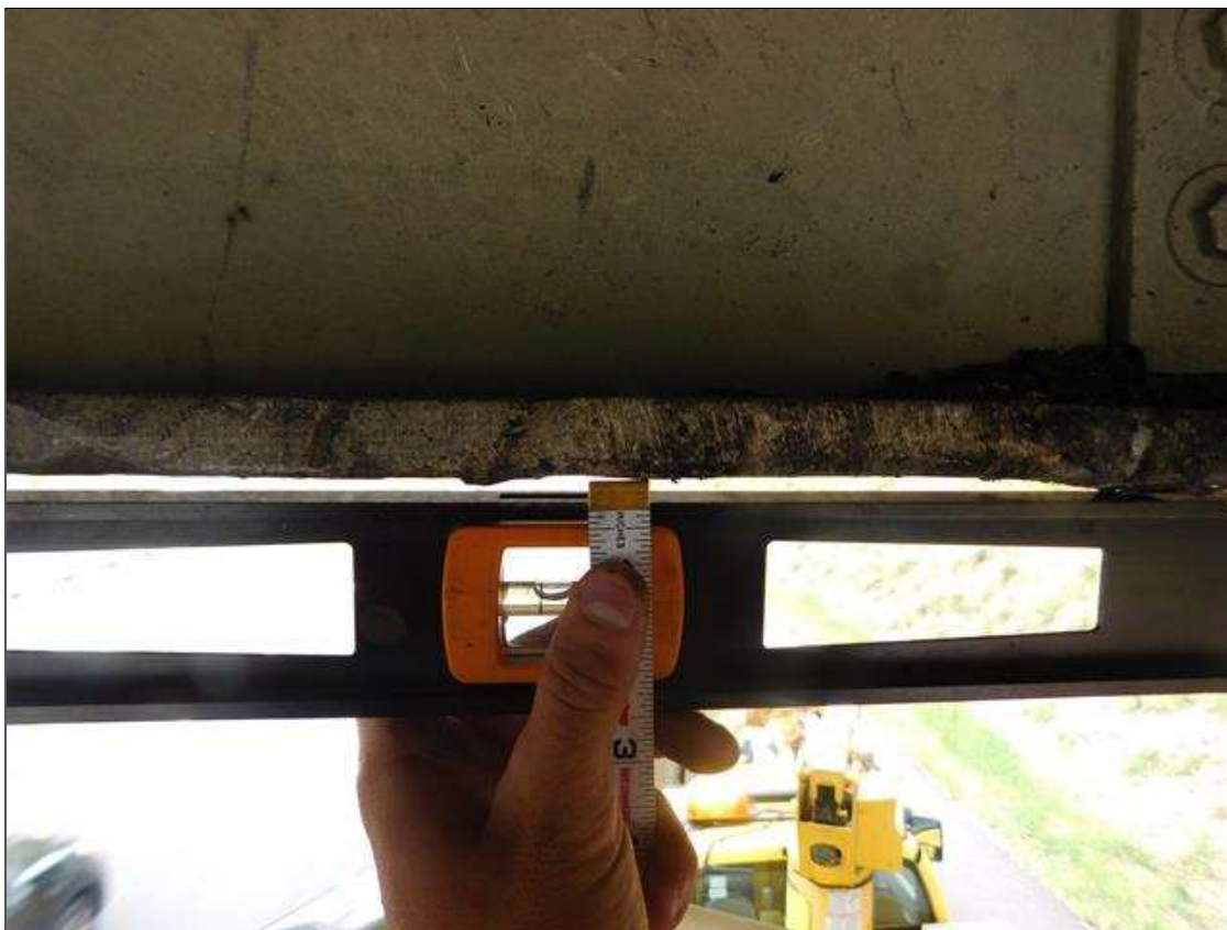
Span 3 Beam 2: BEAM 2 SPAN 3 DEFLECTED UPWARD 1/2" AT POINT OF IMPACT FOR A LENGTH OF 5'
