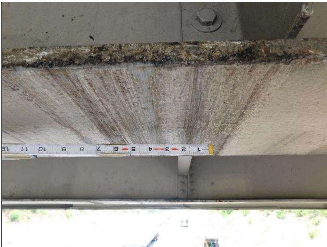
Span 3 Beam 3: BEAM 4 SPAN 3 HAS SCRAPES TO BOTTOM FLANGE AT 16.917' FROM INTERIOR BENT 3 FOR A TOTAL LENGTH OF 2'
