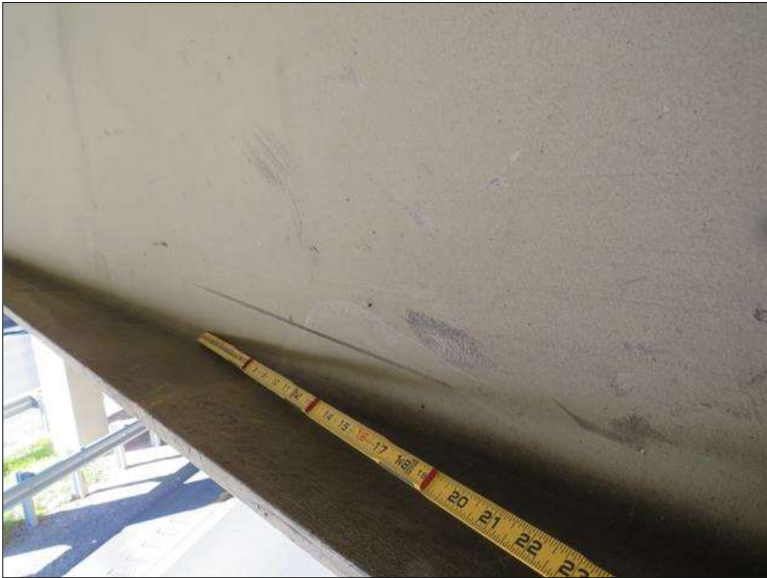
Span 3 Beam 10: SUPPLEMENTAL INSPECTION IMPACT DAMAGE 2021: 1 indentation 1" long x 1/2" deep at 18'-8" from int. bent 3 . scattered scrapes along the web .
