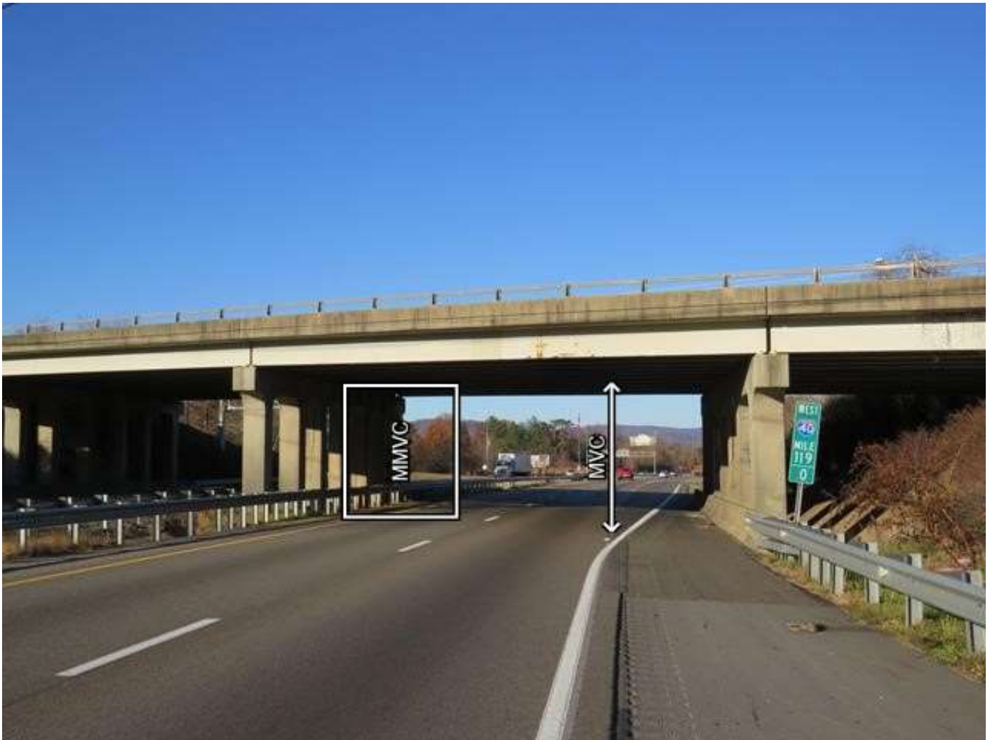
LOOKING WEST CLEARANCE
